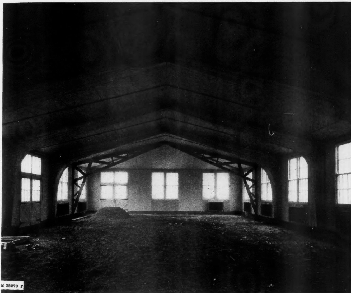
Interior new plywood building of the Laboratory, showing glued arches. Span is 46 feet, walls 12 feet high, ridge 19 feet high. The two trusses in the foreground are built up solid, the third is of double I-beam section and the fourth an ordinary timber truss.
