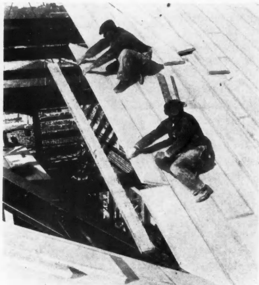
Laying structural gypsum plank
