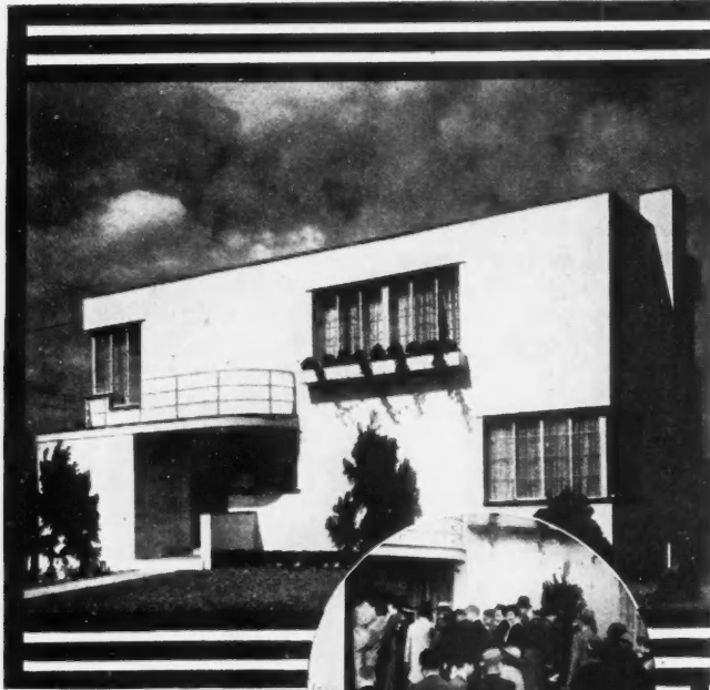
"The Home of Tomorrow" built by the Yonkers Housing Committee under the auspices of the Chamber of Commerce. Concrete masonry walls, portland cement stucco exterior, and concrete-joint first floor with joists exposed to give beam ceiling to basement play room.
