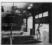
Showing lubritorium type construction, with hi-lift tracks, which raises the door over the hydraulic lift. Used by Shell, Sinclair, Goodyear and other major companies. companies.
