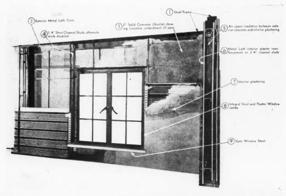
Photo of Demonstration W a 1 I showing s t e e I frame, plastering channels and metal lath.
