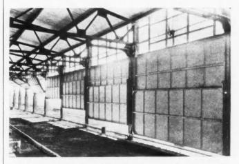
ABOVE: The building of Pier 88, New York, for docking the "Normandie" showing some of the 192 Kinnear steel bifolding doors having a total length of 3880 feet. They range in size from 18 to 37 by 18 feet and required 350 tons of steel panels and 700,000 pounds of counterbalancing weights. Special safety locks protect workmen from this crushing load if the chains should break.
