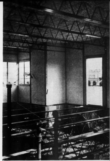
INTERIOR VIEW of Motohome showing rock wool insulation at ceiling held up by chicken wire. Walls are of 2½-inch thick panels made of cane fibre insulating board, with cement asbestos exteriors and interiors which form the finished surface when panels are put in place.
