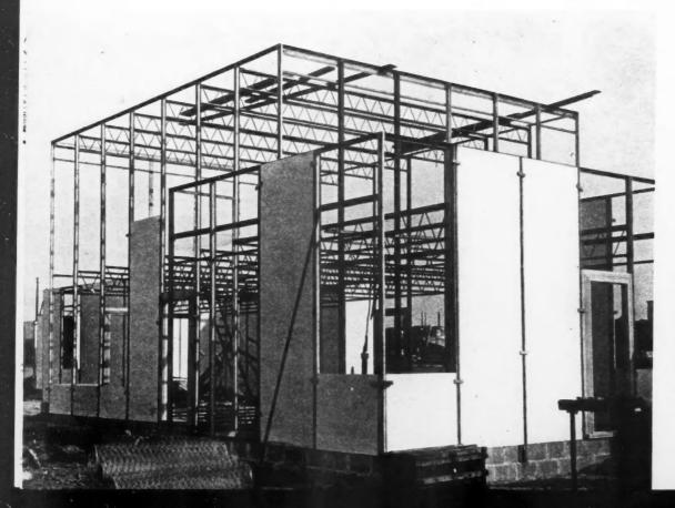
VIEW of two-story Motohome at Boston photographed July 12. Lightweight frame is erected and standard 2½-inch thick panels set in mastic. Wood frame door is shown being placed at right. Exterior joints are covered with aluminum strips.
