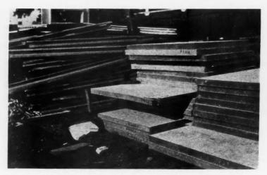
A PILE of Motohome wall panels delivered on job at Boston. Panels are made of four 1/2-inch thick sheets of cane fibre insulating board cemented together with 1/8-inch layers of cement asbestos on outside and inside of panel.
