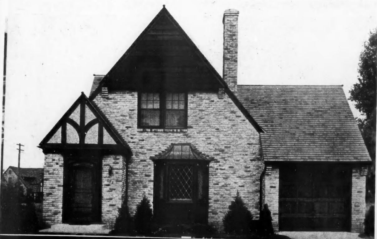
ATTACHED garage at Appleton, Wis., equipped with National Mfg. Co. hardware; Herman Hoepfner, Architect; Fred Hoepfner Sons, Builders.
