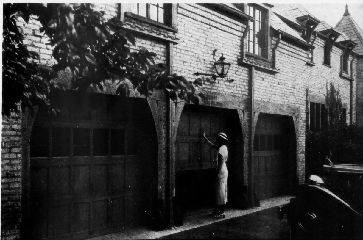
KINNEAR'S "Rol-Top" doors on Columbus, O., residence; R. G. Hanford, Architect; Petzinger & Schlepfi, Contractors.
