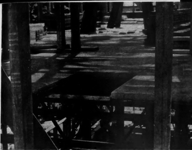
STRUCTURAL GYPSUM FLOORING on Metalumber joists.
