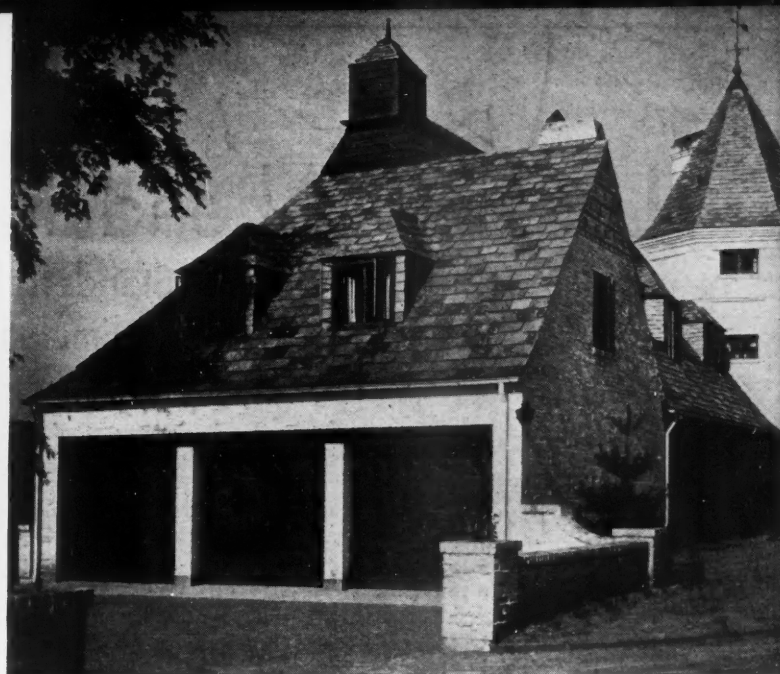
INDIVIDUALIZED design is featured in this triple-door garage in Cincinnati, Ohio; Standish Meacham, Architect. "Overhead" Door Corp. equipment was specified and used, proving entirely adequate to control these heavy doors.
