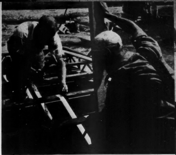
STEEL BAND bridging is nailed in place.
