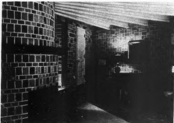
GLIMPSE of circular living room, showing central fire place and radial ceiling beams of concrete.
