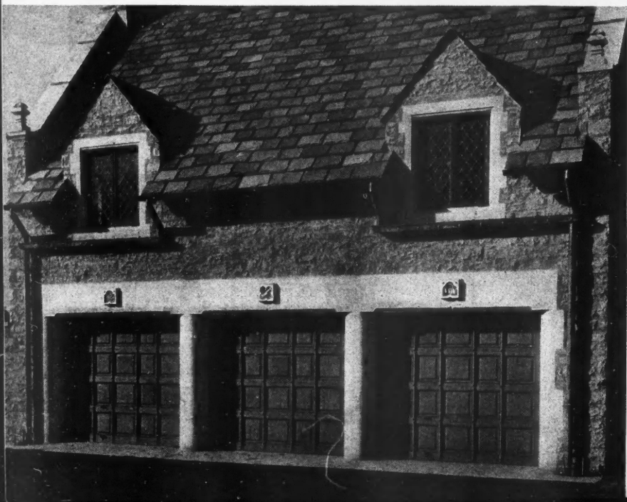
TO left, example of richly paneled garage doors suitable for costly residence. These doors furnished by Kinnear Manufacturing Co. Tetzinger and Schlepfi, Columbus, O., contractors; Benham and Richards, of Columbus, architects.
