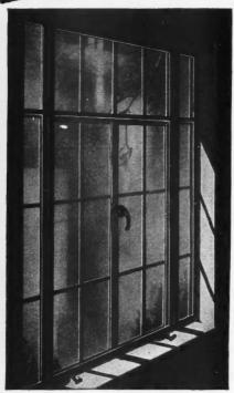
Photograph above (right) shows Fenestra double steel window. Vertical Section (left) shows inner window with tilt-in sill ventilator.
