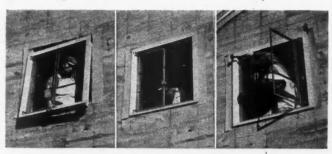
Above, the window with casing and outside trim attached as illustrated below is lifted through the prepared opening from the inside, pulled into place from the outside, plumbed and nailed.
