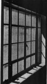
LEFT: Air-Conditioning Window as installation appears from interior with both casement and Tiltin sill ventilator closed; casement handle protrudes through circular aperture, fitted with rubber seal.
