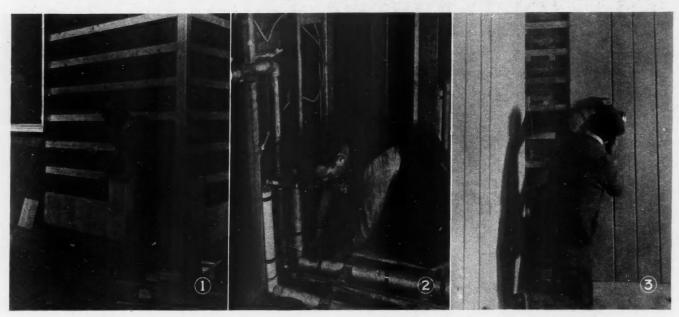
THREE CONSTRUCTION SHOTS on triple-insulated house: (1) Applying asbestos weathered shingles which are fireproof, need no painting; (2) applying pre-shrunk wool-felt pipe covering over hot and cold water lines; (3) bevel plank insulating board in random widths, being applied in basement recreation room.
