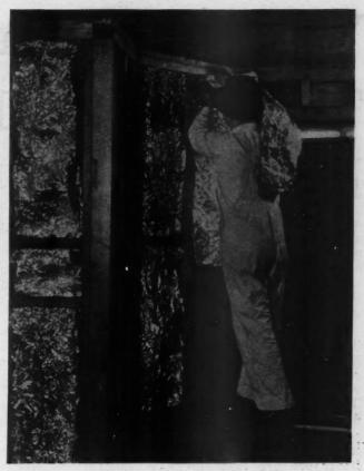
MANNER of installing crumpled aluminum foil into the walls of a house for insulating purposes.
