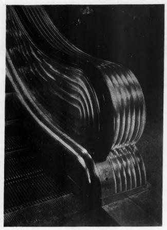
CLOSE-UP view of a well executed escalator rail. The metal has been finished by the Alumilite process.
