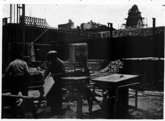
POWER EQUIPMENT was a great factor in the speedy construction of the Chicago World's Fair. Here is a scene during construction of the English Village in 1934, showing use of a popular power machine with band saw attachment, which more than paid for itself on this one project alone.
