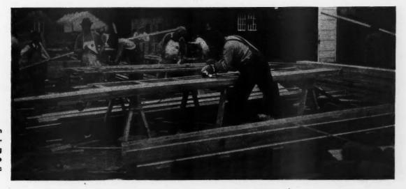
CONCRETE form building involving extensive heavy cutting is done much more cheaply with electric power.
