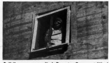
Building paper applied. Fenestra Casement lifted through the opening and installed from inside.
