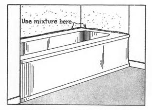
PLASTIC mixture used to fill crack above tub.
