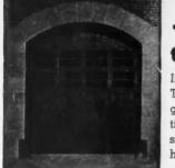
V-grooved Ro-Way Door designed to conform to architecture of building.
