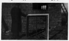
Fenestra Casement and Casing with outside wood trim in place ready for installation.
