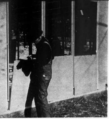
WORKMEN assembling wall panels to steel frame, House No. 2 on Purdue University Housing Research Campus. Cold weather interfered very little with this operation.
