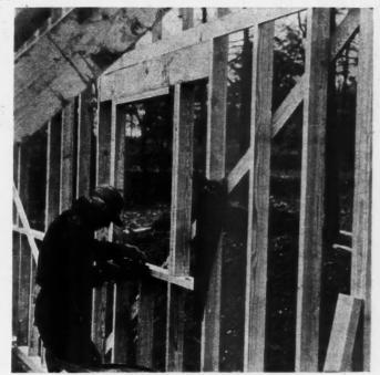
WORK under way on House No. I on the Purdue University Campus, the Housing Research Project. This house, by J. Andre Fouilhoux, architect, is of insulated wood construction with flat roof.
