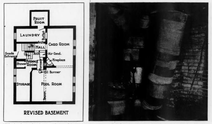
LEFT, plan showing how furnace and air-conditioning unit adjoin chimney. RIGHT, a view of basement Cinderella before the transformation.
