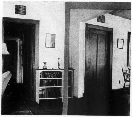
FIGURE 3. A gravity warm air system twelve years old with the trunk above a false ceiling in the hall.
