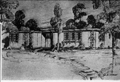
HOUSE No. 2 of prefabricated asbestos cement and plywood panels on a steel frame; constructed by General Houses, Inc., Chicago; Architects Howard T. Fisher and John A. Pruyn associated; construction details and floor plan on this page, photo of construction activity on page following.
