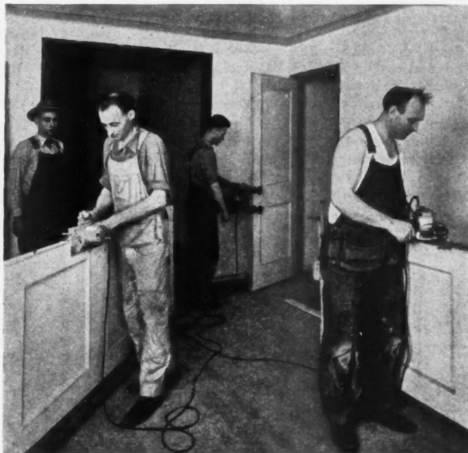
A door being fitted and beveled with a Carter Power Plane.
