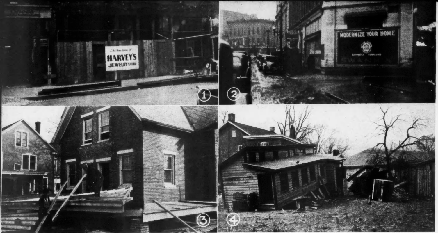
No. 1—The owner of this building in Johnstown is rebuilding 5 new stores. No. 2—Swank's hardware store at Johnstown after the flood. The modernizing sign was completely inundated. No. 3—Flood water stood 4 feet deep on the second floor of this Hancock, Md., house so that the porch floated and later came crashing down. No. 4—A hencoop that went astray.
