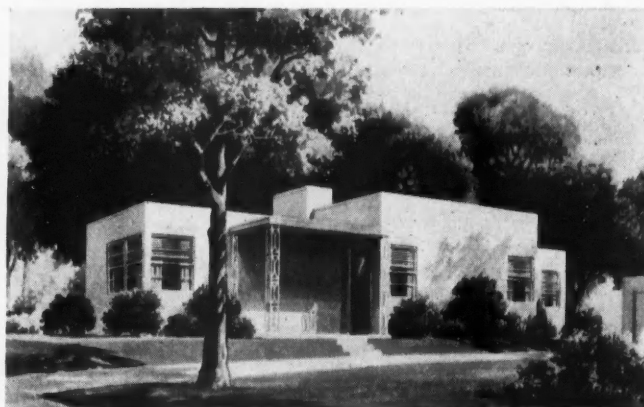
ONE of new modern designs added to Steel Buildings' line.
