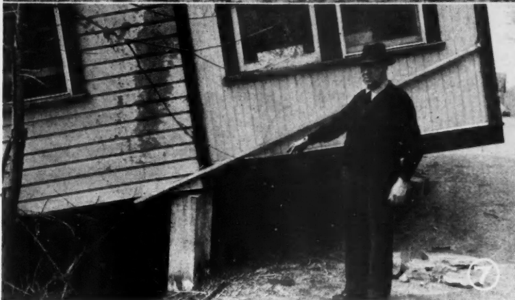
No. 5—This Williamsport, Md., garage was delivered free. No. 6—One of the several hundred store fronts on Johnstown's Main Street. No. 7—Contractor Ernest Miller of Williamsport points out how concrete pier was carried along with this building, which is resting a block from its original site. No. 8—Main Street in Johnstown two weeks after the flood.
