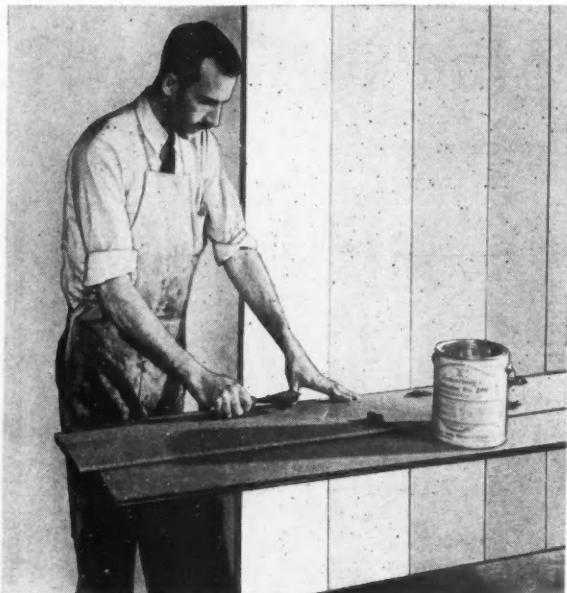
WORKMAN applying Temlok De Luxe with special adhesive.
