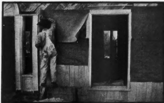
Sisalkraft being applied—"Without holes, without rips or tears"
