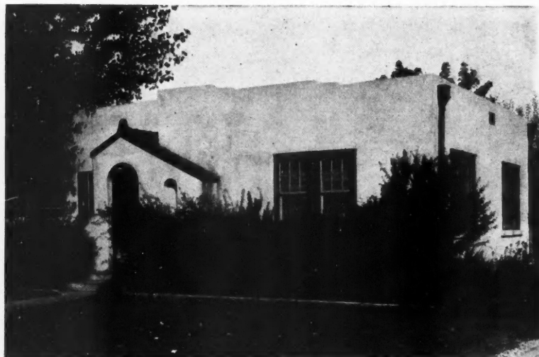
ONE OF THE completed houses built by W. C. Austin is his own home shown above, a good example of the type job he is doing.
