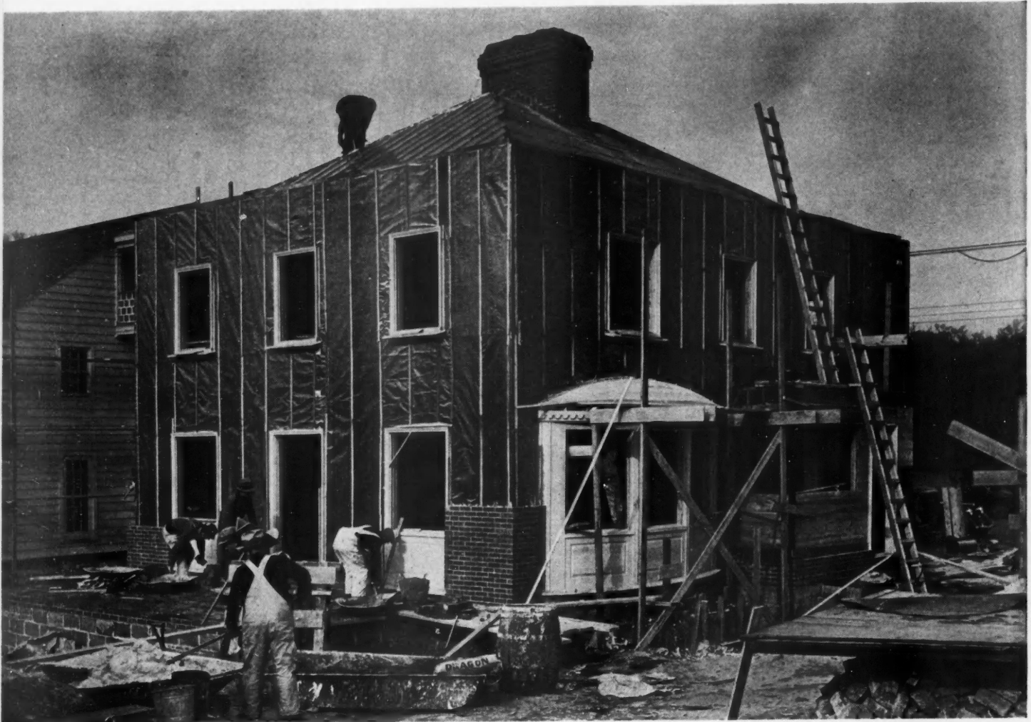
COPPER-Armored Sisalkraft enclosed the Westchester County Model Home of brick veneer construction. Concrete was delivered to the job ready-mixed.
