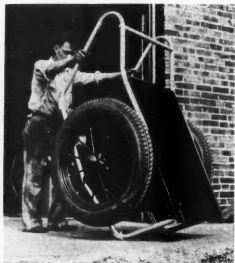
DUMPING is assisted by forward set of legs on new concrete cart at right.
