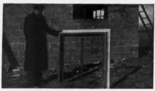
Fenestra Casement and Casing with outside wood trim in place ready for installation.
