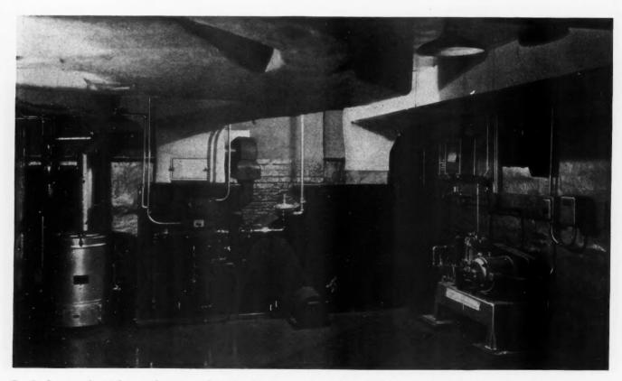
Fig. 3: Basement layout for complete air conditioning. Same type unit as shown in Fig. 1. Incinerator at left. Recording instruments on right hand wall.
