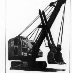
ALL-PURPOSE excavator of high tensile steel for weight reduction and greater strength.
