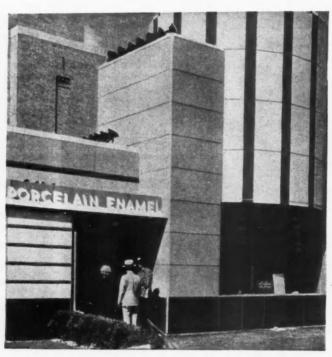
FERRO Enamel Building at Great Lakes Exposition in Cleveland showing exterior surfaces covered with Plymetl panels.
