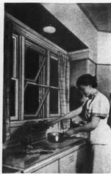
LEFT: Washing Jiffy-Kleen windows is done safely from inside. Right: Sash tilted for ventilation keep out rain and snow in bad weather.
