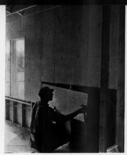
WORKMAN applies the I inch Lok-Joint lath for plaster base and sound deadener on all inside walls and partitions in Insulite home.
