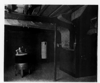
BASEMENT of the Droesch Model Home, showing installation of General Electric NEWSPAPER advertisements of the model home, such air conditioner. House has 12-inch concrete foundation, 3 by 8 floor joists supported on steel beams.
