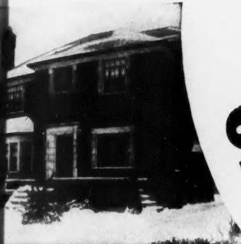
DETROIT, MICH.: Julius Nachman, builder, lives in this house he built. "I have found these systems by far the most satisfactory. When the temperature dropped to 6 or 7 below zero we didn't even know it was cold."
