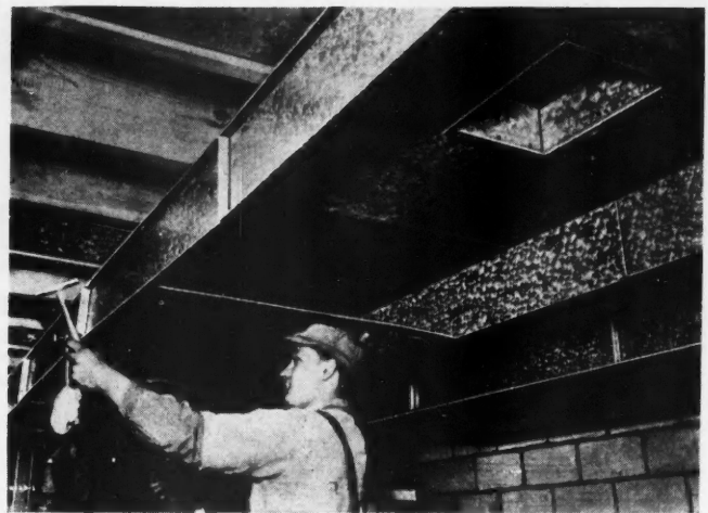
WORKMEN installing air duct system using stock parts.
