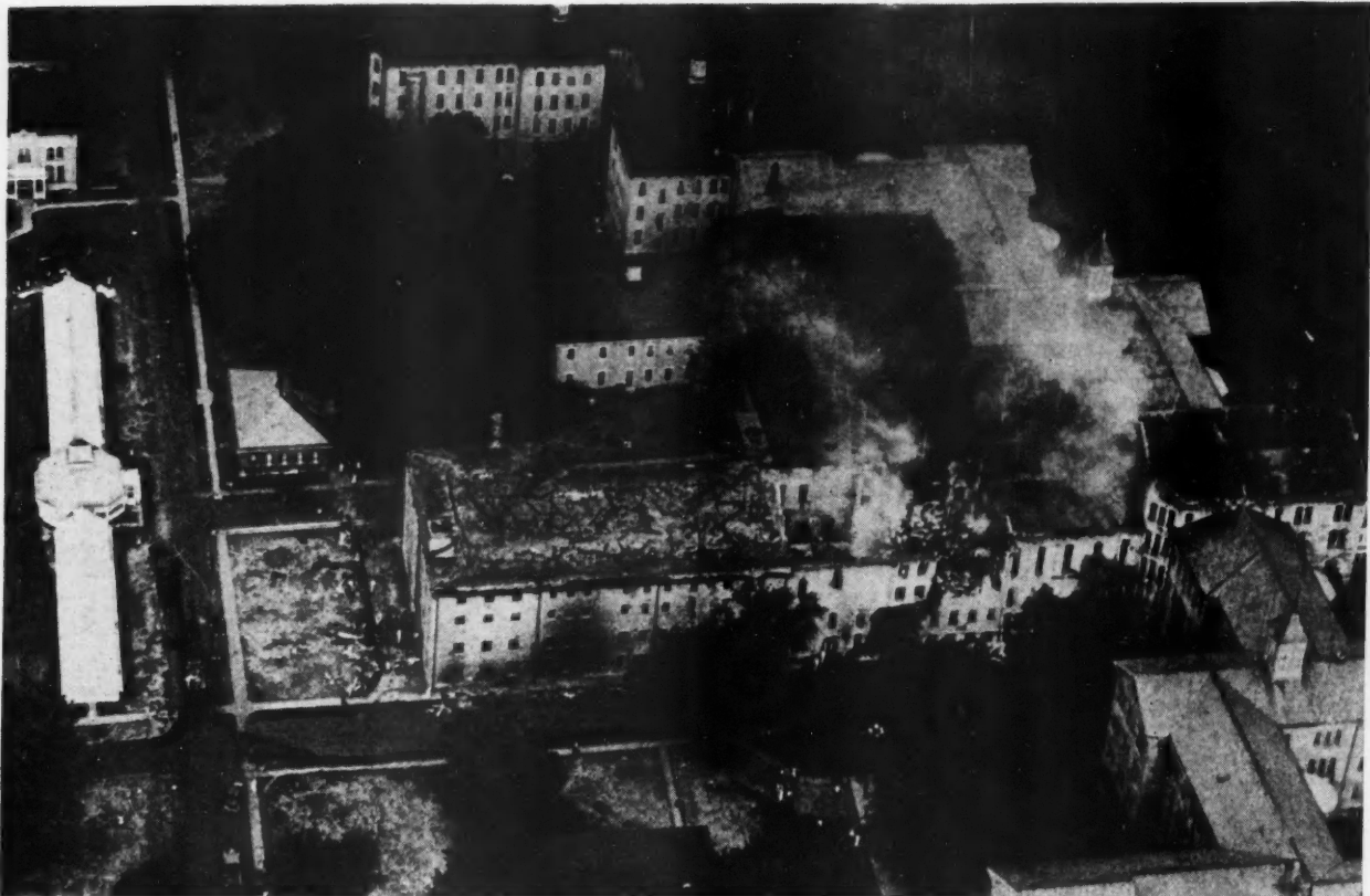
Fig. 3—Fire at a mid-western state hospital. Building in center foreground with roof burned off was saved because its floors were of fire resistive open web steel joist and concrete slab construction. Adjacent buildings not so protected were consumed.
