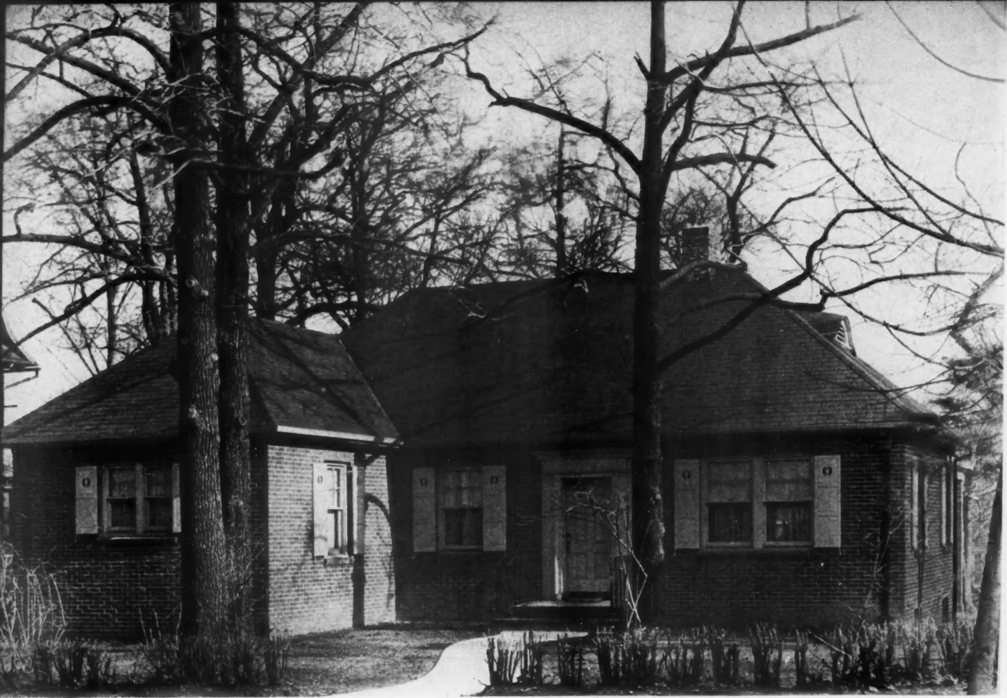
THIS STATEN ISLAND home was built among lovely trees without damaging or disturbing them.
