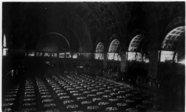
UNION Station waiting room being used as banquet hall.
