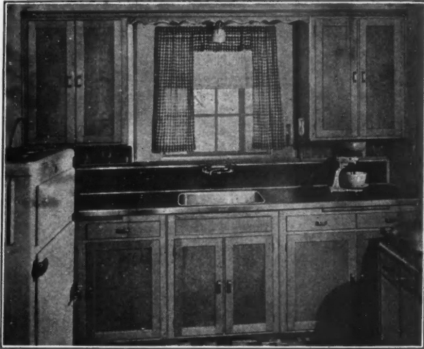
Kitchen Cabinets topped with Tracy Perma Sheen Deluxe Linoleum Sink having an Enduro stainless steel bowl.
