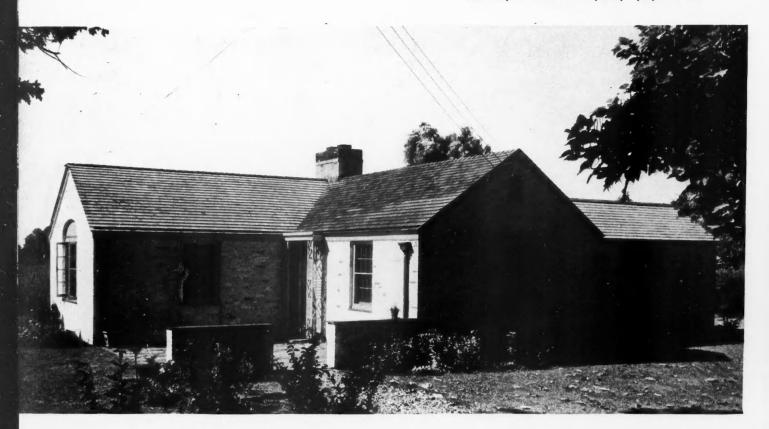
THE SIMPLE details of this entrance give life to an otherwise bare corner. Walls are of second-hand brick, painted with oil paint. Roof is of red cedar shingles. Outside trim is painted cream color.
