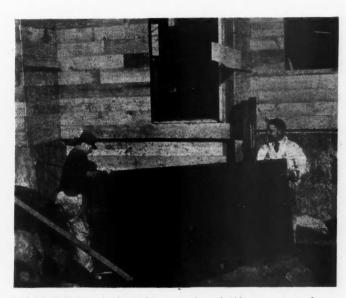
LARGE SHEETS of plywood are used in building concrete forms. These are used over and over and greatly reduce cost of form work. High quality, 2,000-lb. concrete is achieved by water-cement ratio.
