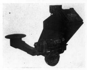
PATENTED "dial control" automatically supplies the right amount of both air and coal in this Kol-Master stoker, made by Paragon Kol-Master Corporation, Oregon., Ill.
