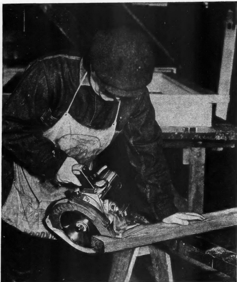
SLANT CUTS and compound mitres are done easily, quickly and accurately with the power saw saving time and money.
