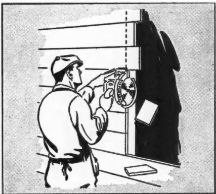
FIGURE 4—Swift work in trimming openings.
