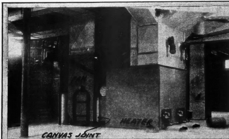
FIG. 2 MORE AND MORE ARE THE INSTALLATIONS OF EFFICIENT, RELIABLE, WELL CONTROLLED AIR CONDITIONING SYSTEMS. WITH THE ADDITION OF COOLING THIS PLANT WILL HANDLE BOTH WINTER AND SUMMER LOADS. (TAKEN LOOKING TOWARD PLAYROOM.)
