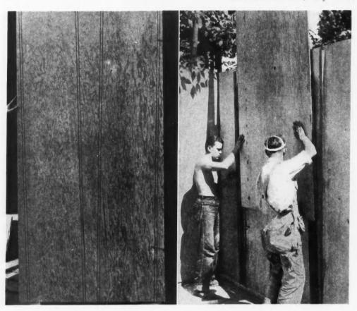
STANDARD size Douglas Fir 1/2" plywood panel, showing the grooves into which ribs will be fitted and glued. In using 1/4" plywood the ribs are glued directly to the face without grooving, and short horizontal stiffening ribs are added. To right: Sliding an interior wall unit into position. Exterior and interior units are identical, but those for the interior are inverted, to interlock with the exterior.
