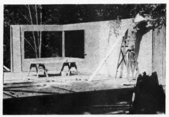
SHOWING how walls are erected. The far corner was started with a window opening and then continued with regular wall units.
