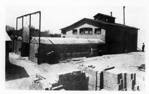
RIVERSIDE Dunbrik Plant; Production building, steam curing kilns and storage yard. loor
