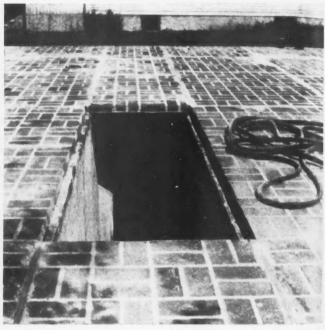
REINFORCED brick panels over full basement, supported with I-beam. Small opening at left hand for hot air register. Floors are terrazzo ground, polished and waxed. Larger opening, stairway opening to basement.
