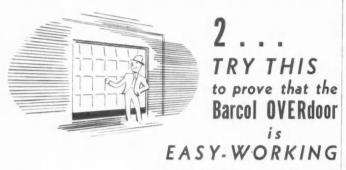
Release the latch, and lift the door! See how easily and smoothly it operates . . . Note how little effort is required to open it. Then look toward the stop strips . . . see how the closing action keeps the door free and avoids sticking. Look at the tailored "twin torsion" counterbalance springs, the ball bearing rollers, the direct-connected cables . . . all important factors that reduce operating frictions and insure easy, long-life operation.
