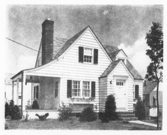
TODAY'S value at \$6650. Compare this with 1929 house on preceding page by the same builder, Realty Associates, Inc., and designed by Benj. Driesler, Jr. It is built on a 60' by 100' plot in a New York suburb, and contains 7 rooms, poured concrete foundation. wood-burning fireplace, scientific kitchen, Venetian blinds, and a wealth of modern detail. The rooms are large. There are two tile baths in the house. The price: \$6650 including land.
