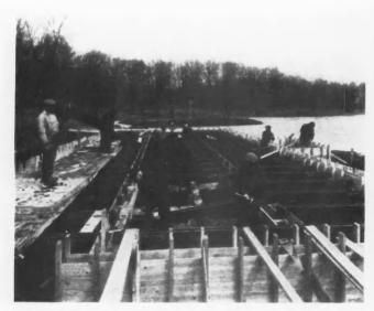
HOLLOW steel sections being laid across foundation wall forms ready for laying of White-Steel slabs.
