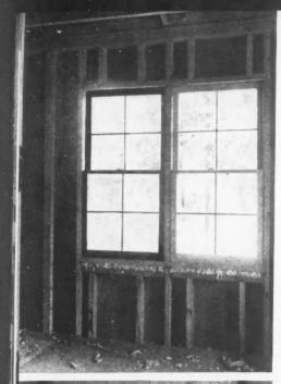
LEFT: View of framing around opening which has a lining of weatherstrip and serves as jamb and head. Note sash balances and narrow "Furstix" mullion; alue strips have been applied to joists and the stud at far left.
