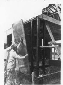
NOVEL building methods tested as workmen erect metal wall panels on the "Copper House," Washington, D.C.
