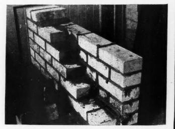
Figure 2—Workmanship A, showing complete filling of joints
