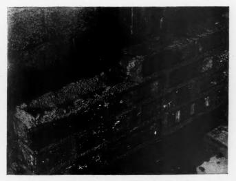
Figure 3—Workmanship B, showing furrowed bed joints and buttering of bricks for head joints
