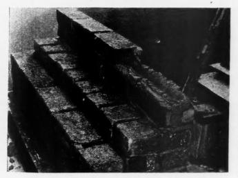
Figure 4—Workmanship B, showing poorly filled joints
