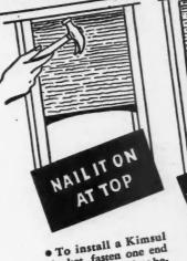
blanket, fasten one end to the header or plate beto the neader or plate be-tween studs, then draw the free end down, like a roller shade, and nail to sill.
