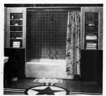
**LACK OF LARGE-UNIT TILING** a decade ago ran up the cost of vitreous walls. Decorative wall boards were developed in an effort to reduce the cost of covering kitchen and bathroom walls. In 1929, Johns-Manville manufactured and sold a decorative board consisting of a sheet of flat transite covered with a lacquered finish. It was fireproof, easy to clean, and attractive in appearance. The finish, however, was not as durable as the 1937 product.
