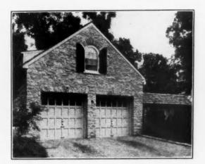
THE ORIGINAL OVERHEAD DOOR gave birth to a new idea in closing openings—a door tight at top, bottom and sides that occupied no valuable space and that could be made to fit any opening.
