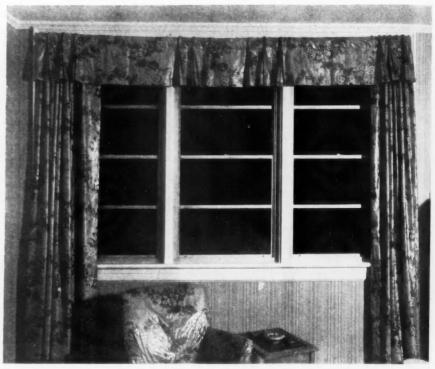
EASY operation, weathertightness, and complete elimination of upkeep expense are among the features of this Kawneer Light Sealair Window.
