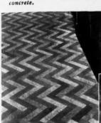
Blocks are also easily nailed or applied in mastic to soft-wood sub-floor.
