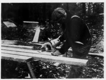
POWERFUL electric hand saws such as this reduce sawing costs more than 50%. They are an important factor in making possible more rapid construction of homes, higher labor productivity and lower costs.
