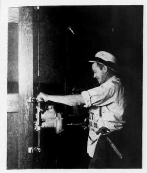
SLOW AND EXPENSIVE hand mortising of doors is being replaced by the electric mortising machines. With the mortiser above, 45 perfect mortises can be cut per hour—a tremendous reduction in the time and cost of this operation.
