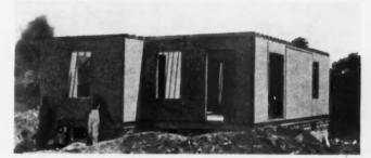
SHOWING ERECTION of a small home by precision-built methods using Homasote board in sheets up to 8 x 14 feet.
