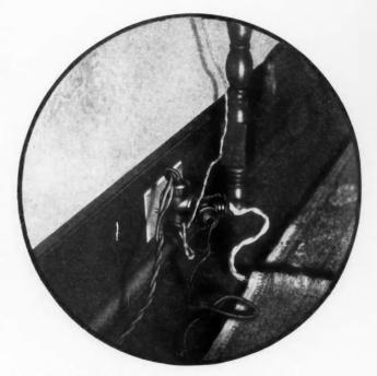
NO MORE OF THIS—The modern home must provide for enough convenient places to plug in electrical devices and equipment without such accumulation of dangling, dangerous wires seen above.
