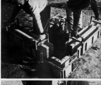
STEP 2. The mix is thoroughly tamped and form is ready for removal after concrete is properly placed.
