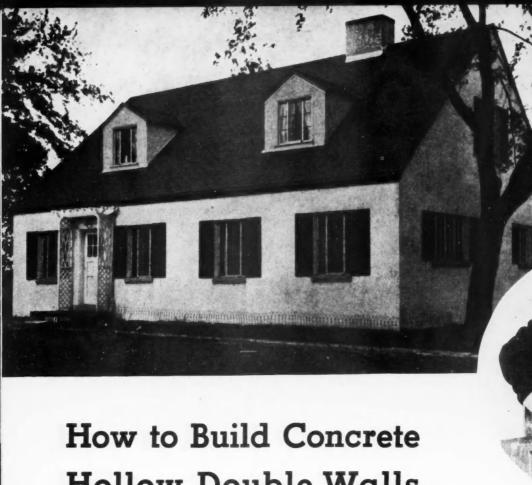
LEFT: House in East Troy, Wis., built of monolithic concrete placed with hollow double wall form system.
