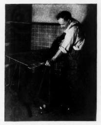
Straight cuts can be made with ordinary hand saw, preferably a 9 or 10 point saw. The sawing should be done on the finished side.
