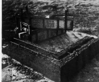
STEPS 3 and 4 (below at right). Cross ties and horizontal reinforcement are laid and forms set for second course. Pins lock forms together.
