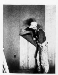
THE straight-edge felt is tightly buttjointed, thereby providing an absolutely smooth surface for the paper.
