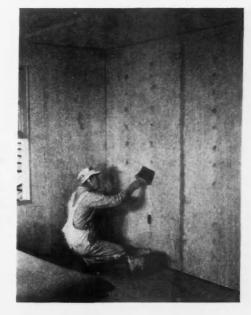
SIZING the plywood with wall-paper paste before hanging the felt assures better a dhesion. Joints and nail holes are filled with crack filler and smoothed with a sand-paper block.
