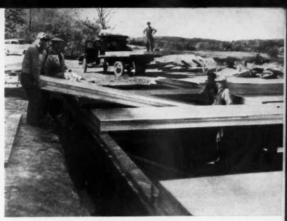
PHOTO above shows floor panels being assembled on foundation at Forest Products Laboratory Plywood house.
