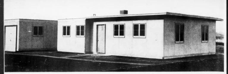
THE new prefabricated plywood panel house at Madison, Wis., designed and built by the engineers of the Forest Products Laboratory. Photo shows all panels in place and house completed.
