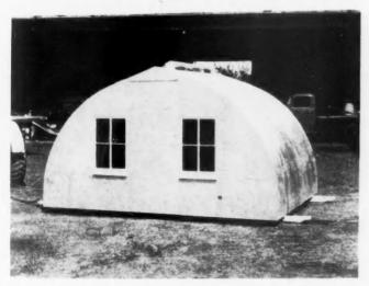
POULTRY broader house using laminated bent rafters and plywood panels weigh less and are stronger than when built of natural lumber.
