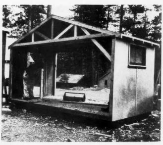
PORTABLE bunkhouse developed by the U. S. Forest Service for rangers in the Tieton Mountains. Sections consist of Douglas fir plywood walls, floors and roofs with simple trussed rafter construction. Units are bolted together on the job when these portable bunkhouses are assembled.
