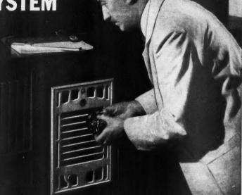
THE Arco Thermo System uses a new principle of heat distribution in rooms. With a new unit concealed within the walls of every room it brings to homes instantaneous circulation of warm air, without the disadvantages of ducts.
