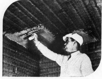
**INSTANT BOND.** Overhead work is speeded up and 'plaster droppings cut down...resulting in definite savings in materials and time, and Steeltex Type A can be easily bent to form true, sharp corner and ceiling angles with *continuous* reinforcing.
