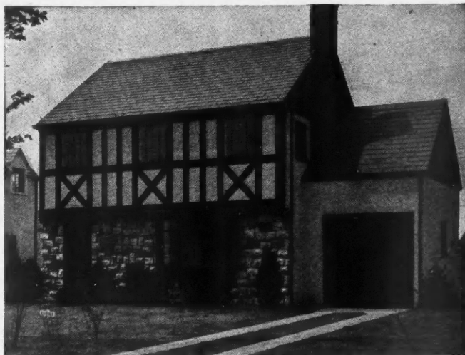
Stucco made with Atlas White portland cement was used in finishing more than half of the homes in this beautiful development. Atlas Gray cement was used for the house foundations and roads.
