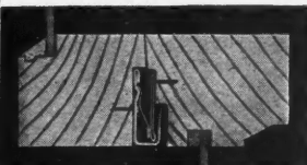
Section Through Check Rail. Note the NEW three-piece weatherstrip with concealed nailing and spring leaf metal-to-metal contact.
