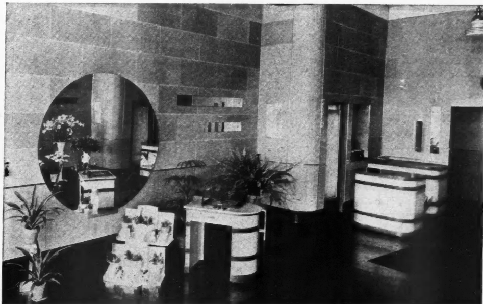
REMODELED florist shop in San Francisco uses fiber board and glass effectively for modern interior.
