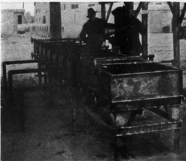
VIBRATING Table (above) with glimpse of electric vibrating motor; below is shown gang of joist molds on table; filling is either by hand or spouted gravity feed.
