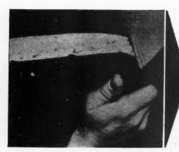
Cut end of Balsam-Wool showing Spacer Flange\* as it fits over framing members to form a tight, wind-proof joint with air spaces front and back. Lath is eliminated. Easier, faster, positive application is assured with the staple hammer. Balsam-Wool cannot sag or settle.
