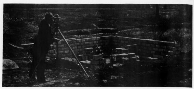
WITH SEVERAL FEET YET TO GO, foreman establishes exact level points with pencil mark at each corner. Masons then measure up from pencil marks. Result is a finished foundation true within one-eighth inch. Saves masons' time and eliminates delays in leveling sill.
