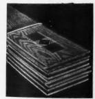
Endless Lumber for sheathing is tongued and grooved on ends and edges. Since the boards interlock, pieces do not have to be joined over framing members. This simplifies application. diagonal Much sawing is avoided and strong, tight walls are secured.
