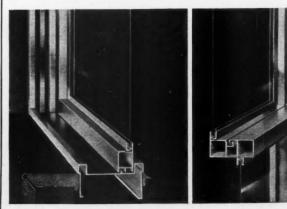
CORK TILE . LINOWALL . ACQUITICAL CEILINGS | CROSS sections of Kawneer all-aluminum sash showing construction
