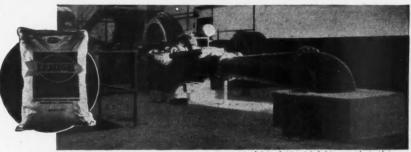
When the city of Manchester, N. H., installed a new pump at the Water Works, speed was essential. Therefore in making concrete alterations and the new pump foundation, Lehigh Early Strength Cement was used. The new pump was set in place within 24 hours after pouring. C. L. Ahlgren was the Engineer for the city.
