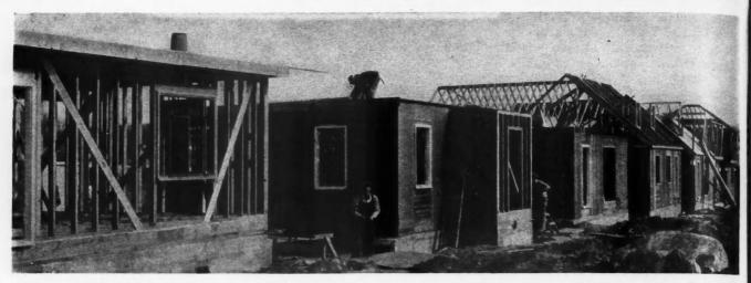
CONSTRUCTION VIEW of a row of low-cost Gross-Morton homes at Jamaica Estates, Long Island. Large sheets of asphalt and aluminum coated Vapor-seal sheathing are used on exterior walls.
