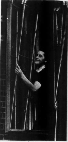
A HOME with modern prefabricated doubleglazed sash can be "window conditioned" in a few minutes. The extra, insulating sheet of glass is fitted into a special recess in the sash.
