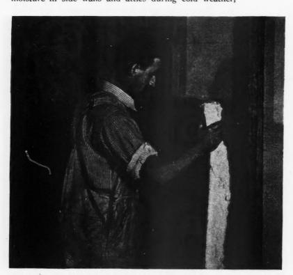
MINERAL WOOL in batt form simplified installation. The latest improvement is the addition of vapor-proof paper backs. All forms of insulation now are available with vapor seals, to eliminate condensation in sidewalls and attics.
