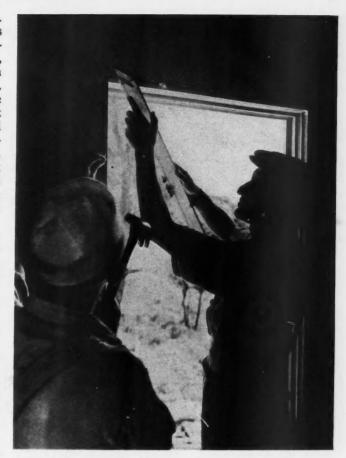
INSTALLING FACTORY CUT TRIM on one of the Westminster Ridge houses of Lee Perry, White Plains, N.Y., builder. Windows and frames are also delivered to job completely primed, weatherstripped and ready for quick installation.
