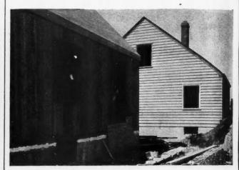
A MILLS HOUSE ready for siding over Celotex sheathing; note cement grout to seal at foundation line and tight fit around Fenestra sash.
