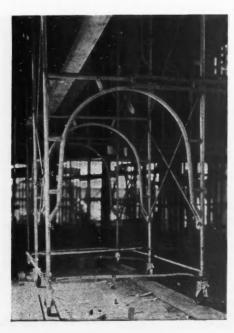
NEW TYPE movable steel scaffolds in use inside one of the buildings at the New York World's Fair. Scaffolds are of sectional style, quickly erected or taken down. A. L. Hartridge Construction Co., builder.
