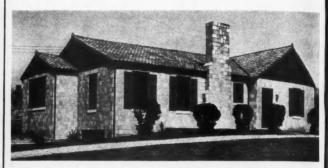
HOME of Dunstone ashlar construction, Knoxville, Tenn. Mat glazed cream, buff, tan. Sizes used: Standard Dunbrik 21/4x33/4x8, Dunstone (double brick) 8x8x21/2, and Dunstone (triple brick) 8x12x21/4.
