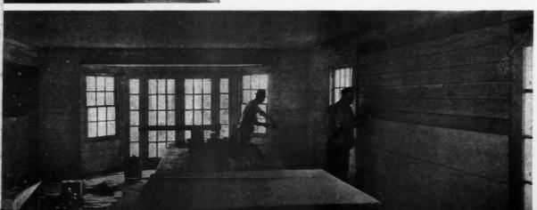
LEFT: Horizontal boarding applied over studs or furring gives a good nailing base for panels and allows joints to be placed without regard to framing. Tendency to buckle is also eliminated; crating lumber is satisfactory for this job.
