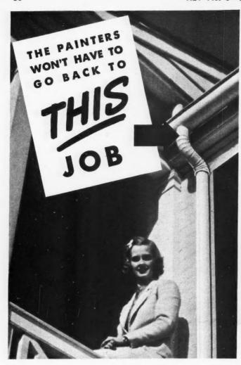
The gutters and downspouts are made of Armco galvanized PAINTGRIP Sheets, and were painted as soon as installed. There was no waiting for weathering. No acid etching either, which eats off part of the protective zinc coating.
