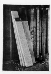
ABOVE—Factory fabricated ducts delivered to job ready for installation. AT RIGHT—Steel door frames and wood window frames delivered on job at Kenwood development of Charles Reis, Riveredge, N.J. Door bucks are steel.
