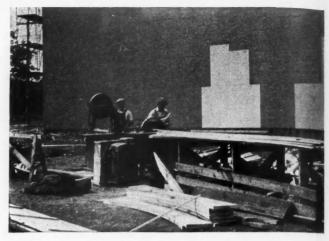
POWER SAW and woodworker operated by compact gas engine in use in construction of buildings at New York World's Fair by the A.L. Hartridge Co. The bandsaw made possible a particularly large saving in the cutting of the circular units shown in the foreground.
