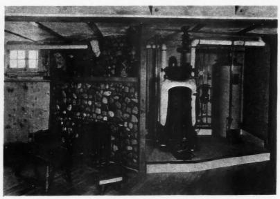
GAS-FIRED boiler and automatic hot water heater. The heating plant in this conversion job has been placed on a white tile platform, raised above the floor level of this unique basement, with its attractive fireplace of field stones, and rustic furniture.
