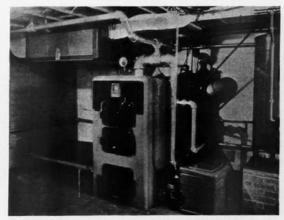
SPLIT-SYSTEM heating and air conditioning plant. A bin-feed stoker fires this boiler automatically. The boiler is connected with a heat exchanger that furnishes conditioned air to most of the rooms above, and is connected to radiators that supply heat to small rooms in which it is inexpedient to install return ducts.
