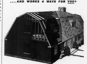
\* INSULATES. MASONITE DUBBLSEAL SHEATHING is MASONITE STRUCTURAL IN-SULATION 25/32-inch thick. It is coated on all sides and edges with a special water-proof asphalt . . . a super-effective barrier against the passage of heat and wind infiltration!
