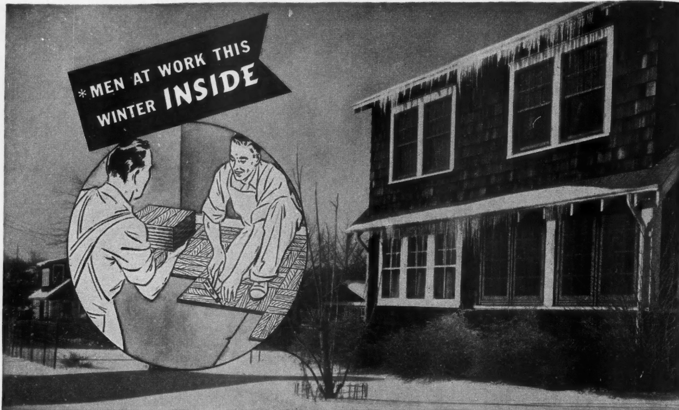
*LAYING NEW FLOORS OF BRUCE FINISHED HARDWOOD BLOCKS
