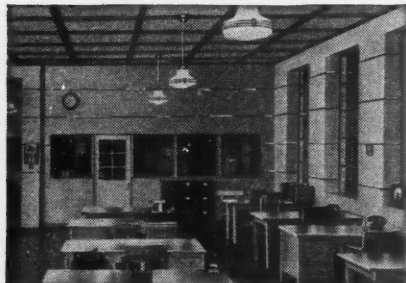
IN OFFICES: —Standard Flexboard assures permanence, presents a pleasant, dignified appearance. On this installation, it was painted to harmonize with ceiling decorations.
