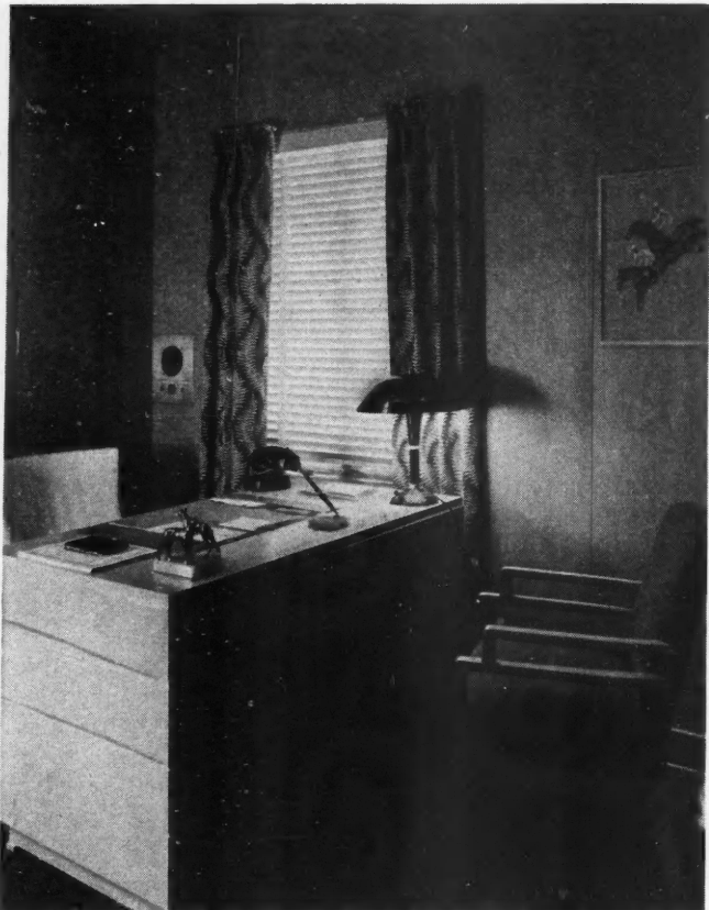
FIG. 5. Here a "Vee" joint is used to good advantage. This illustrates one of the most practical methods of paneling plywood. Architect, W. F. Ruck.
