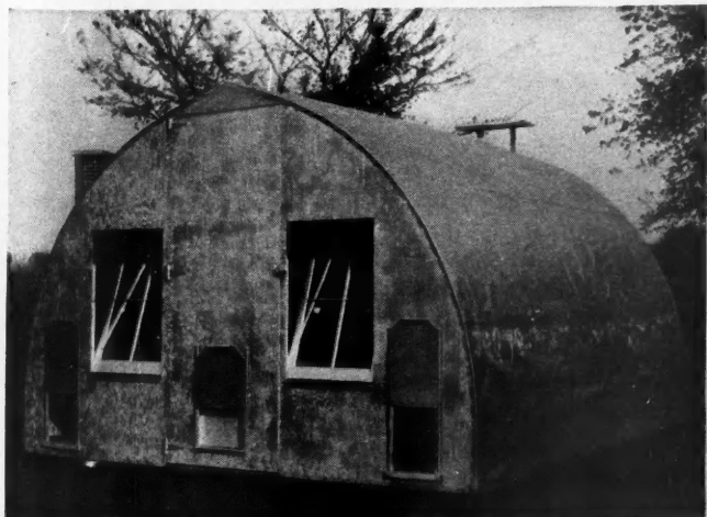
FIG. 14. Poultry house of Douglas fir plywood tested for strength of construction.
