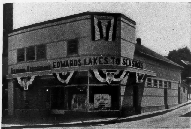
BUS DEPOT in Pennsylvania "covered" with "EXTERIOR" Douglas Fir Plywood. The cut-out letters shown are also of this waterproof plywood product.
