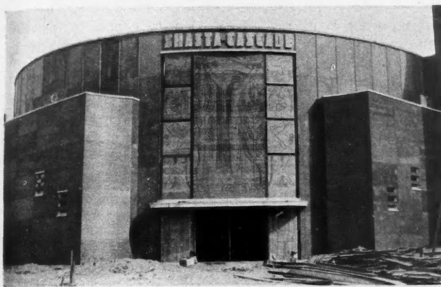
THE BUILDING of the Shasta-Cascade (California) County building cased in "EXTERIOR" type Douglas fir plywood shown before it was painted. In the interiors literally acres of Plywall, the Wallboard grade of plywood, have been used.
