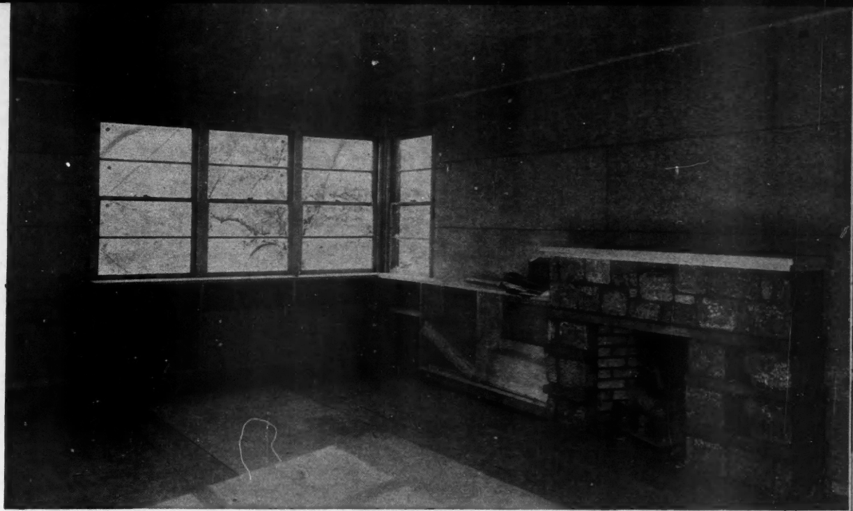
LIVING ROOM of Rosenfield house, showing use of "V" joint with stock 8' x 2' panels. A detailed drawing is given below.
