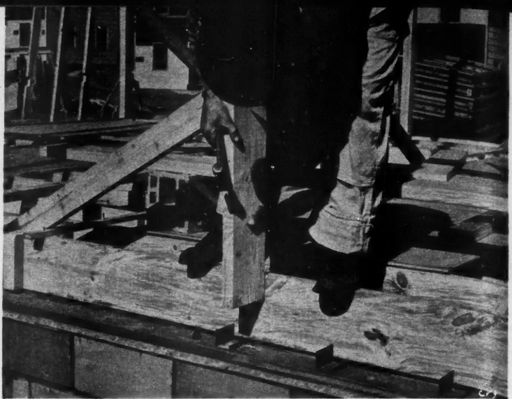
STEEL SILL PLATE and ribbon with nailing flange for studs provide accurate spacing and more rapid assembly. AT LEFT, carpenter is seen nailing steel ribbon notched into 4 x 4 corner post. AT RIGHT, carpenter is seen fitting stud into nailing flange on steel sill plate.
