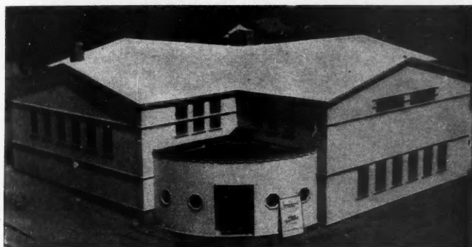
Typical Job, REZITEX on SUPER HARBORD All-Plywood Gym, White Salmon, Wn.
