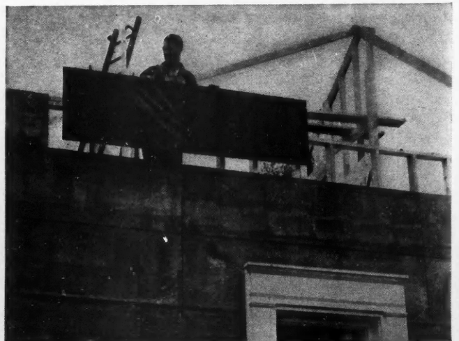
WORKMAN applying new 2 - 8 foot size asphalt-coated sheathing.
