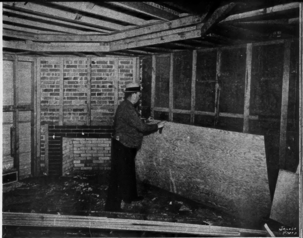
ABOVE: PLYPANEL grade of Plywood being applied to the walls of the recreation room in the basement. As wall covering for rooms of this sort Plywood is a preferred material.
