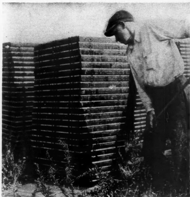
DOUGLAS Fir Plywood concrete form panels ready for oiling and subsequent use for exposed concrete surfaces of the foundations of the 74 buildings in the Buffalo, New York, Lakeview Housing project. As soon as the panels are stripped from the foundation of one building they are cleaned, oiled and taken to another unit.
