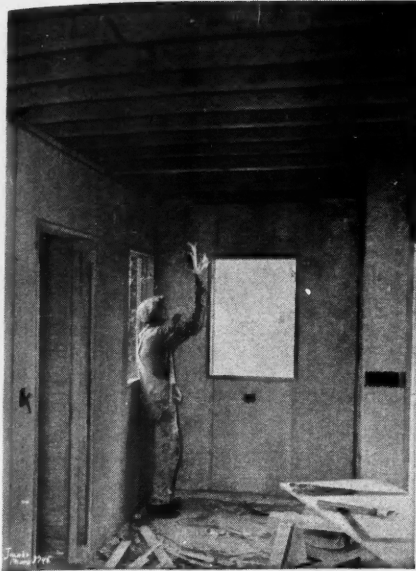
WORKMAN applying PLYWALL, the wall-board grade of Plywood to the walls of one of the bathrooms where it served as the base for tile. In kitchen also it served as tile-base.
