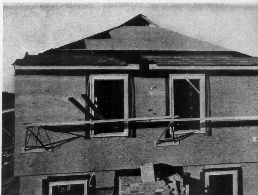
ROOF SHEATHING of 5/16" plywood is used, over which asphalt shingles are laid on 30-lb. roofing felt.
