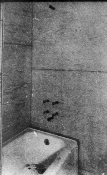
ATH ready for sheet rubber surface.
