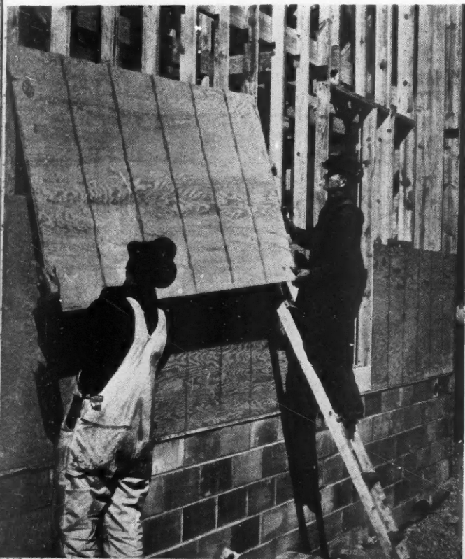
ABOVE—Erecting steel ribbon—the first step in framing Gilbert and Varker houses. BELOW—A crew of two carpenters and a helper completely enclose exterior walls and roof of house with Douglas Fir "Plyscord" sheathing in 7½ hours.
