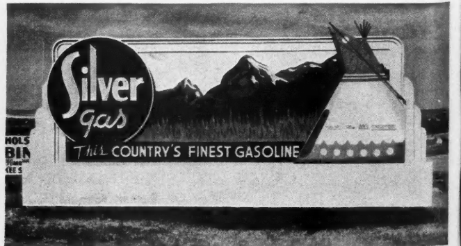
PERMANENT outdoor sign boards form an increasingly large market for the "EXTERIOR" grade of Douglas Fir Plywood. Impervious to the weather, since the glue-line is completely waterproof, many of these sign boards have been in continuous use for several years.
