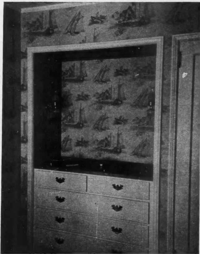
FIG. 11. Wall paper applied to a bedroom built-in. Plywood is now widely used by many builders for closets and built-ins because it is adaptable and workable and will not splinter or warp.
