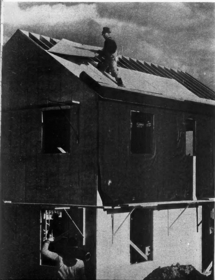
APPLYING 5/16" plywood sheathing to roof.
