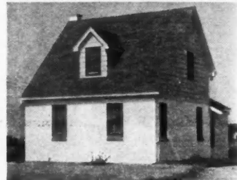
IN the upper view of a Detroit residence in the low-cost housing field, cinder block walls are seen unpainted. In the lower view two coats of Outside Luminall have given the job an intense white covering.
