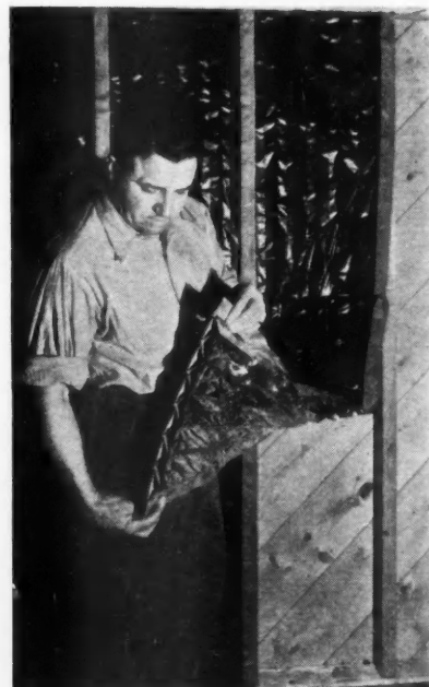
CELLULAR structure of Type 2 Air-Met insulation and application to stud faces is shown in the view at the right.
