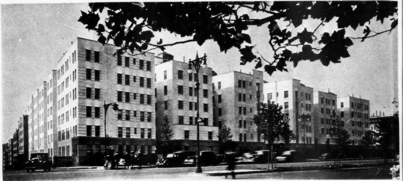
VIEW OF NEWLY REMODELED Roosevelt Garden Apartments in New York City. They were the last word in 1922.
