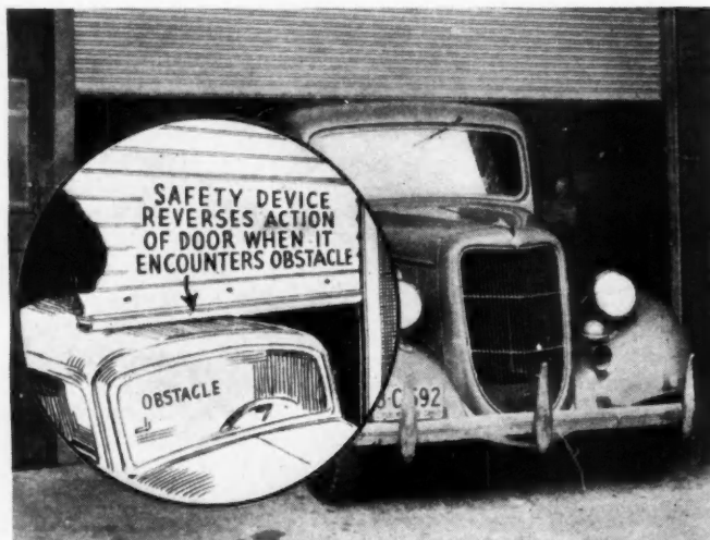
WHEN door strikes obstacle, it stops or reverses automatically.
