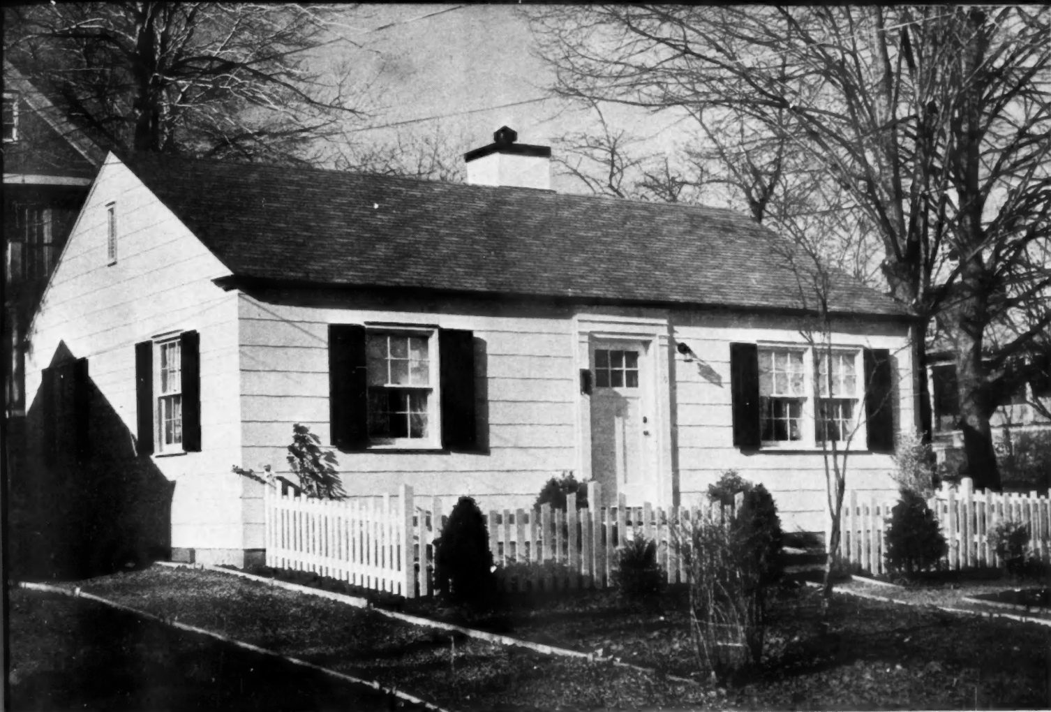
ONE of the compact, 4-room basementless houses typical of the group shown on the front cover, in H & B Corporation development.
