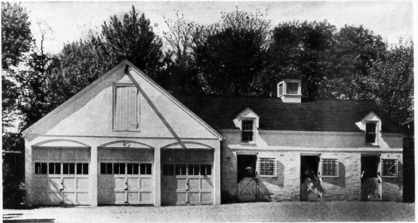
THREE HORSES, two cars and a pony cart are attractively housed in this building on the estate of H. G. Bergen at East Williston, L. I. General character of design would harmonize with any type of Colonial styling.
