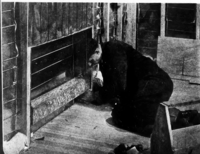
FIG. IX—CONCEALED COPPER FIN RADIATORS are installed (below). Insulation consists of sheet steel forced between the studs.
