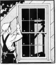
SET UNIT IN WALL Units are set by nailing weathertight wide blind stop to stude, which insures a weathertight joint.
