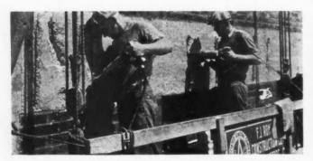
F. J. ROMER COMPANY, St. Paul contractors, saved 75 percent in direct labor cost in cutting out concrete with electric hammers.
