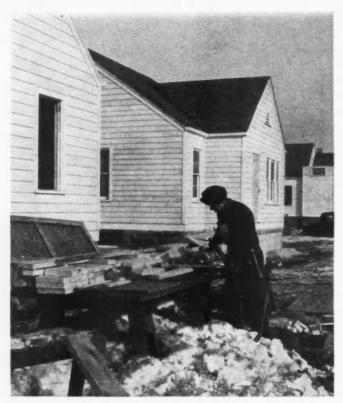
CUTTING of window framing with power hand saw is fast and accurate on Hammond, Ind., project even in cold winter weather.
