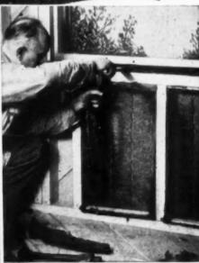
AND EVERY BIT IS USABLE! Even short ends left over from insulating non-standard spaces make ideal caulking
