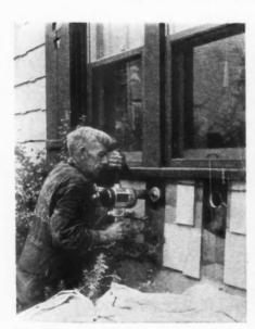
drill is used on walls to cut holes up to 31/2". er floor machines at edges and in corners. and refinishing on wood or other materials.
