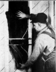
2 NOTE HOW CONVENIENTLY it can be worked around wires, pipes, etc.! As flexible as a blanket, obstructions in a wall cause no difficulties when insulating with Kimsul...
