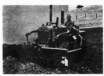
BULLGRADER mounted on a tractor speeds the work of Contractor Ted Oliveira, Lafayette, Calif., on the excavation for the basement of Orinda Public School. Backfilling and grading are also simplified.
