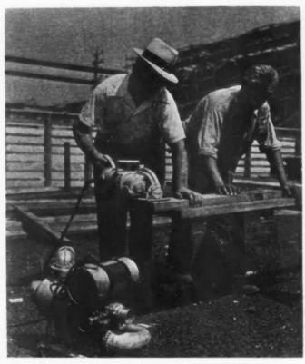
PORTABLE GENERATOR supplies current for this electric hand saw on New York World's Fair job; electric supply is usually available.
