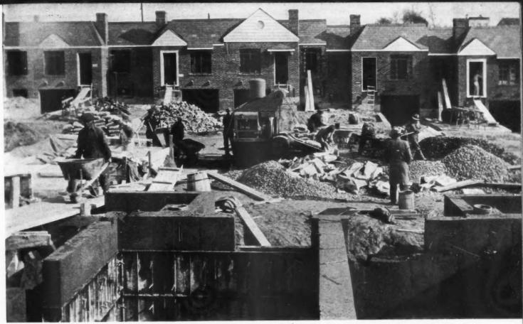
A MODERN CONCRETE MIXER, steel forms, rubber-tired wheelbarrows contribute to lower cost, better quality concrete at Green Park Homes, a successful row house project near Forest Hills, L. I. BELOW Lightweight Safety Saw with plenty of power, equipped with duplex handle for convenience in any position; cuts 2-inch dressed lumber. Scaffold brackets are time and material savers.
