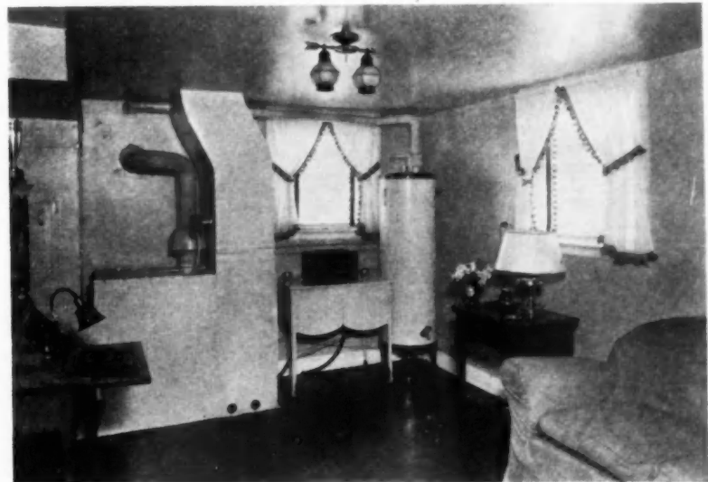
HEATING and hot water equipment blends attractively with color plan in this basement living room where separate space for such items was not available.
