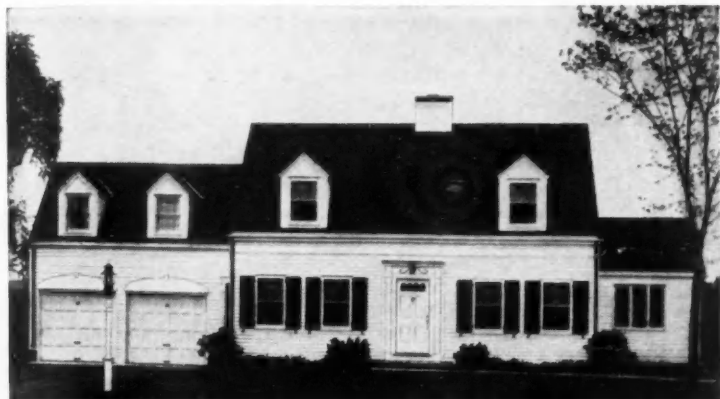
R. G. BENT, Builder A. RAYMOND ELLIS, Architect, Hartford, Connecticut
