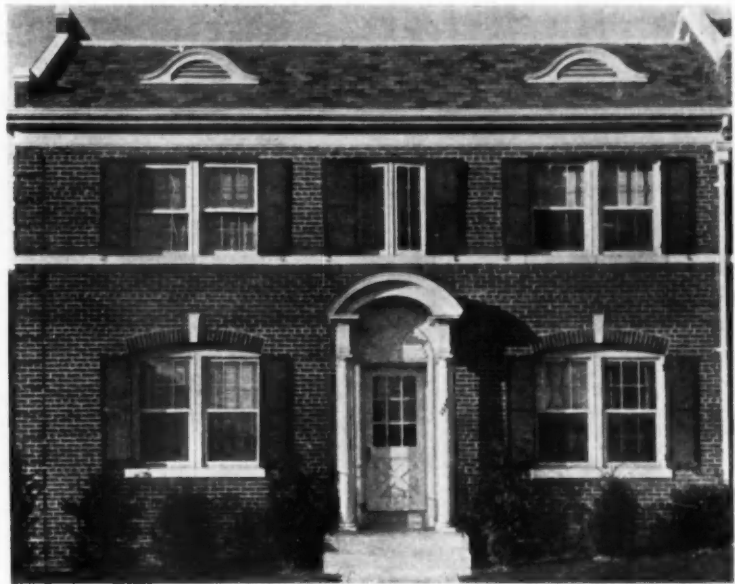
TYPICAL WASHINGTON ROW HOUSE unit which has individual gas heat and hot water equipment.
