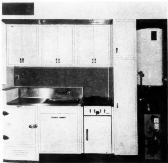
COMPACT PACKAGE-TYPE EQUIPMENT used in modernization work. Includes a gas heating unit and hot water heater with storage tank.
