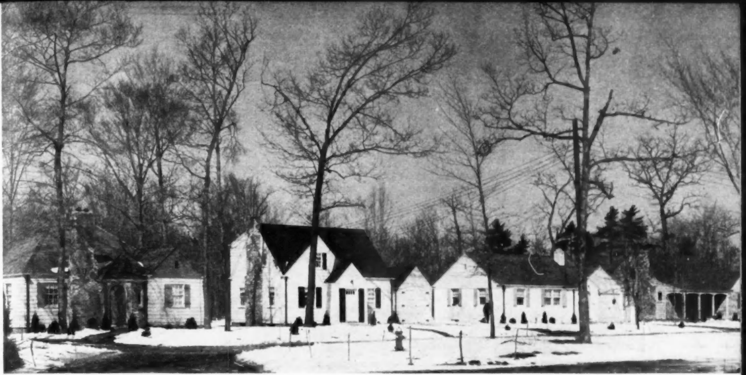
ROLAND COURT—All-gas home community at Cromwell, Conn. August Tobler, builder.
