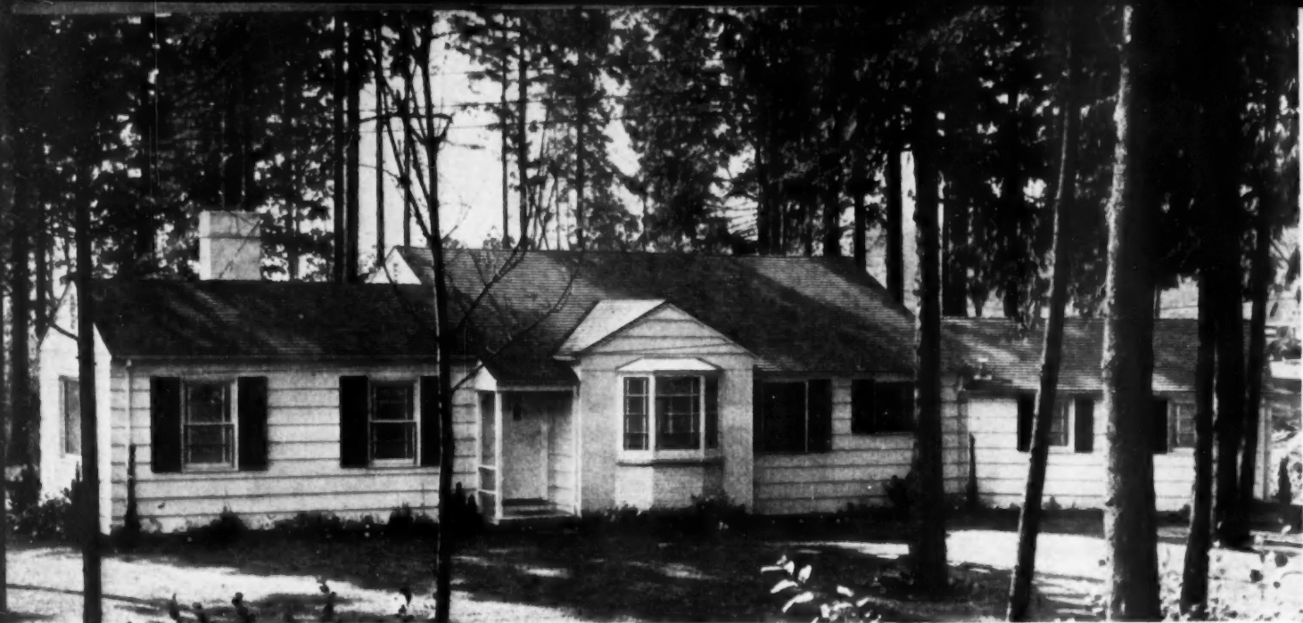
GAS-EQUIPPED MODERN HOME in new Beñz Park, near Portland, Ore., designed and built by J. Wayland Owen.
