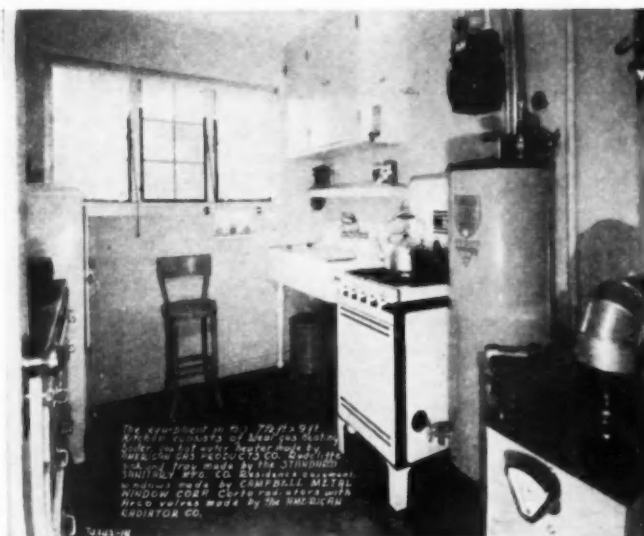
A 7½' x 9' MODERNIZED APARTMENT KITCHEN in which is located an individual gas heating boiler and hot water heater, as well as range, refrigerator and standard kitchen equipment.
