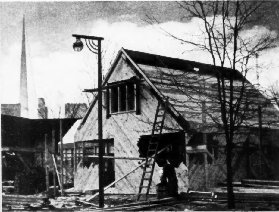
NATIONAL LUMBER MANUFACTURERS' ASSOCIATION home demonstrates new type of economy framing, roof trusses and practical use of plank floors.
