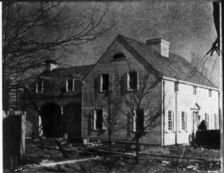
KELVIN AIR-CONDITIONED HOME demonstrates latest in equipment and services. Designed by Electus D. Litchfield.
