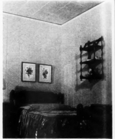
DRY WALL INTERIOR CONSTRUCTION features use of decorative insulating board.
