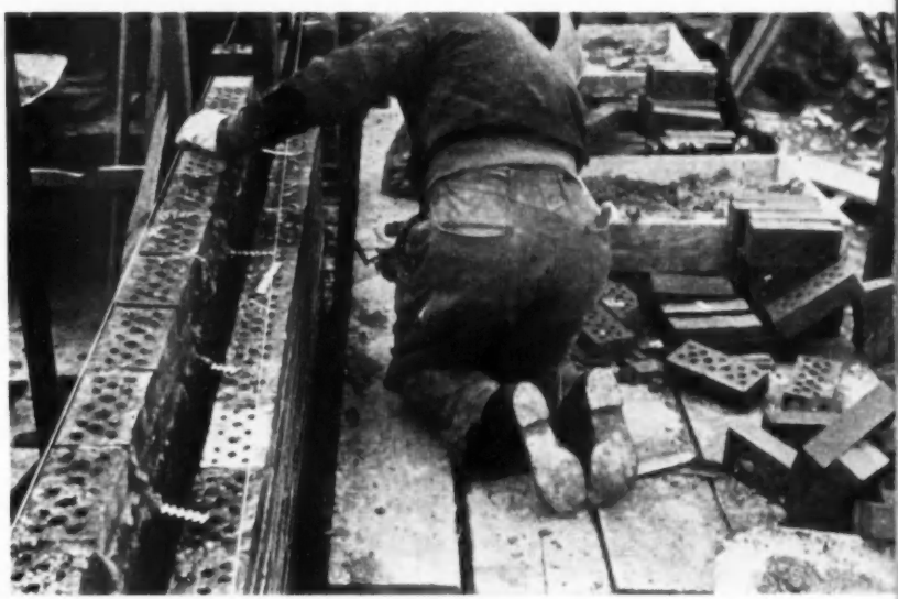
PHOTO ABOVE SHOWS BRICK CAVITY WALL under construction, leaving 2-in. air space that prevents passage of moisture and acts as insulating barrier. Note metal connectors to tie the walls.
