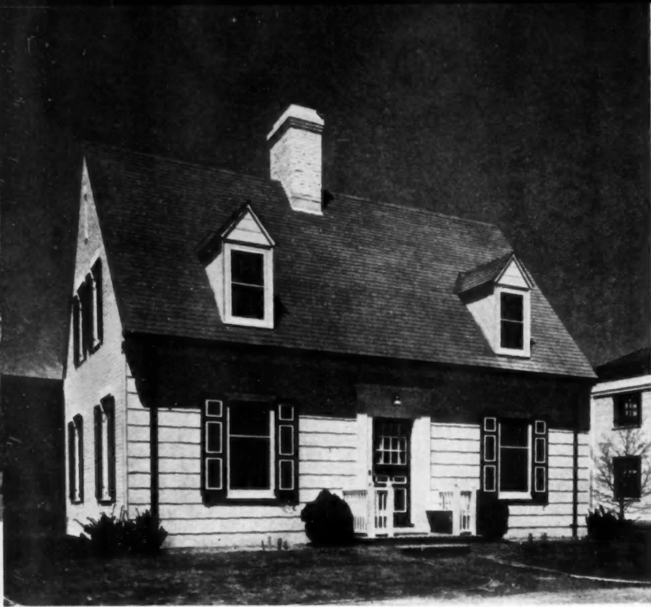
FEATURING shake-textured asbestos wall shingles and Curtis entrance.
