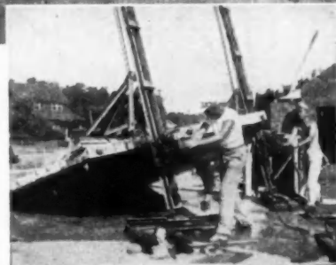
Tilting up wall to vertical position with simple hoists.
