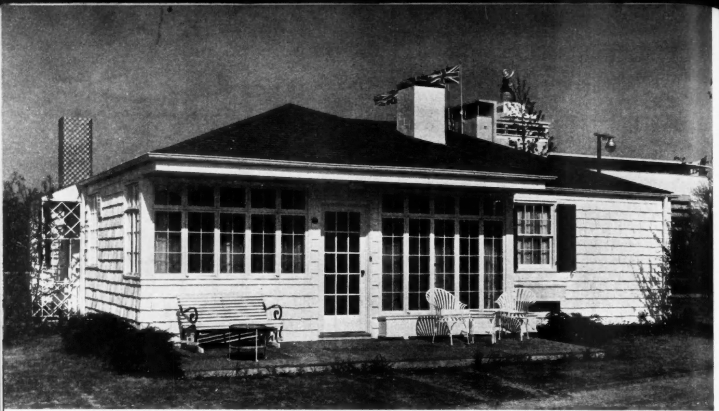
THICK-BUTT HAND-HEWN SHINGLES contribute deep shadow lines and beauty to N. Y. World's Fair House No. 1.
