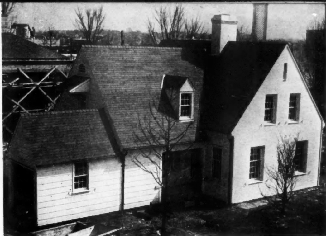
SIDE ENTRANCE to Triple Insulated "Tomorrow Town" house. Roof is of cedar-grained asbestos shingles. Side entrance provides convenient garage connection.
