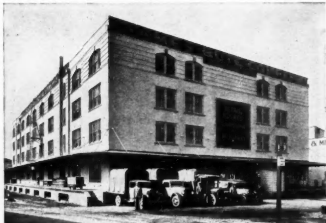
Houston warehouse of James Bute Company, weatherproofed and preserved with a treatment of No. 109 (stone gray) Bondex.
