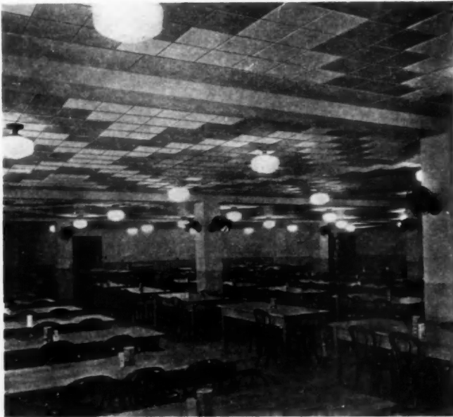
THE ALVIN SCHOOL, of Alvin, Texas, uses ceilings of Armstrong's Temlok De Luxe in white and ash to decorate, insulate, and quiet noise.
