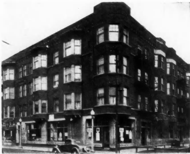
55th St. and Ellis Ave. Building, Chicago, modernized and restyled; 4th story removed, bays torn off; revised floor plan shown opposite.
