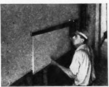
Lok-Joint Lath fits directly to the house studs and makes a smooth, safe, crack-proof base for plaster.
