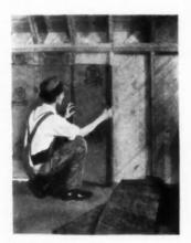
THIS thoroughly insulated McCarthybuilt model home sold a few days after the opening, and is now being duplicated, with a few minor changes. The house is 23'6" x 46' overall, gas heated, and fully insulated with 4" superfelt bats.
