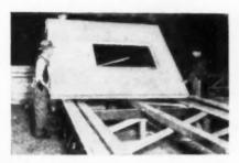
Wall and partition units are framed from working drawings, with doors and windows integral
