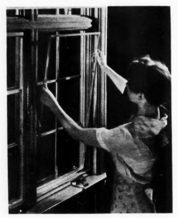
STORM SASH comfort (above) from accurately fitted unit windows. Today this health protection is not an afterthought but is provided in the window assembly as it comes from the manufacturer. BELOW is shown the modern inside storm window for wood casements. Manufacturers advise leaving them on the year round. They're installed in a jiffy. Complete with spring leaf weatherstrip, they swing with the sash.
