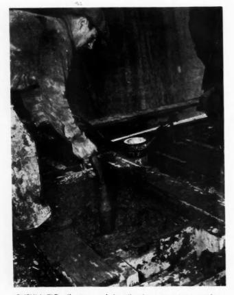
PNEUMATIC vibrator used in vibrating cement to produce a denser mix and assure the complete filling of the forms.
