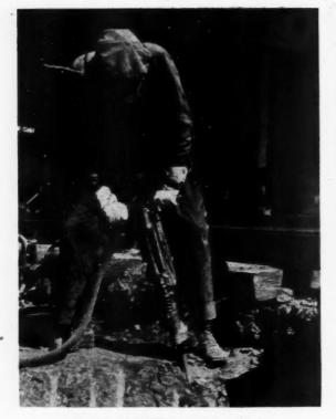
PAVING BREAKER rips up concrete.
