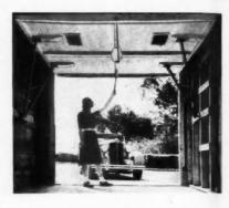
UPPER view, Strand garage door is lowered by convenient rope pull. Lower, view of closed position.
