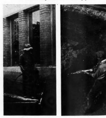
CONCRETE SURFACER (at left) operated by compressed air used on Indiana school. AT RIGHT, pneumatic clay digger speeds difficult digging.
