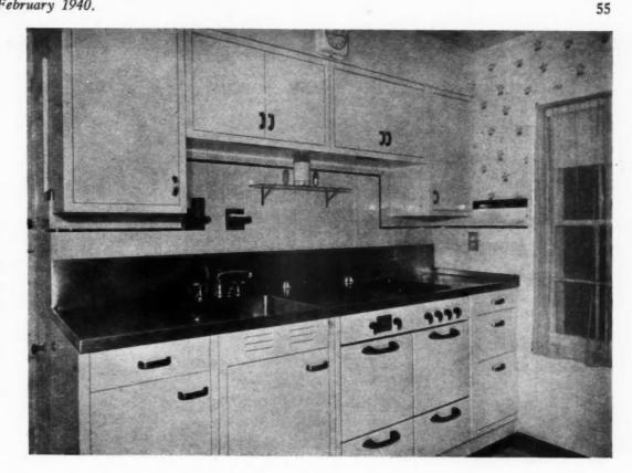
ANALYSIS of the modern gas kitchens submitted by builders from all parts of the country shows a definite trend towards the use of more factory-built, or prefabricated equipment. Practically all have factory-built cabinets which require a minimum of time for installation. An important factor in built-in equipment is that it is eligible for longterm financing under the FHA insured mortgage.
