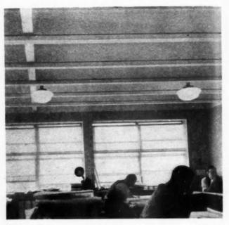
EXPOSED joists in offices of Massena & DuPont, architects, Wilmington, Del. No plaster used on ceiling.
