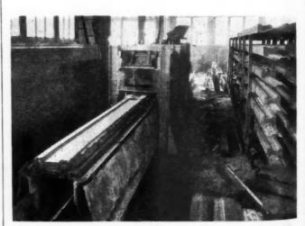
LITH-I-BAR concrete joists emerging from W. E. Dunn machine in Formigli plant, Philadelphia, for U. S. housing project.
