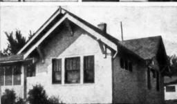
THE top illustration at the left (1) shows a small bungalow just before Nelson resurfacers start work; paint failure due to structural faults is to be remedied (2) with a stucco overcoating.
