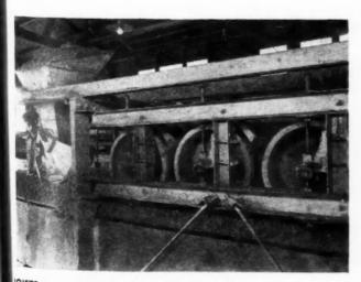
JOISTS are machine rolled under 2,000 lb. per sq. in. pressure.
