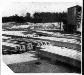
1300 feet of machine-rolled concrete joists on truck
