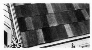
ASBESTOS-CEMENT strip shingles lay flat without warping.
