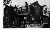
sheathing. On pitched roofs, Fir-Tex sheathing insulates where the greatest heat loss occurs; adds materially to the structural strength of the building, and provides a permanent moisture barrier.
