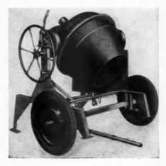
END discharge permits greater efficiency in loading barrows; discharge height, 27 inches.
