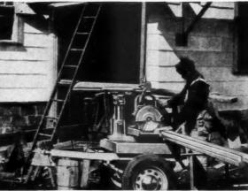
Straight-line production in house building lumber travels from pile directly across work table into house. Saves time and labor.
