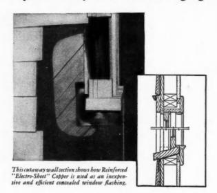
To DETERMINE the relative effectiveness of the various available materials for water- and moisture-proofing, tests were recently conducted on twenty-one different products, five of which incorporated thin sheet metal. The metallic products, including four reinforced "Electro-Sheet" types, were the only ones to prove impervious to water and water vapor both before and after accelerated aging. Such efficiency more than makes up for their moderate extra cost.
