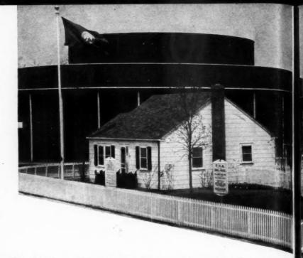
THE \$2,500 house illustrated at left, above, and fully detailed below, is well proportioned and well laid out, with a full basement. The exterior is of asbestos cedar grained siding shingles, and the roof of multicolored asphalt shingles. Interior walls and ceilings are of gypsum board. Hall arrangement is efficient.
