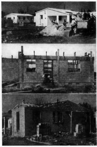
ABOVE at right, construction of Preu houses showing, at top, foundation being poured; center, beam forms in place ready for pouring on top of block wall; and bottom, roof being framed. At left, precast concrete window frame being set into the mesonry wall.
