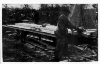
CONSTRUCTION views show, top, 2 by 6 subflooring being laid over 4 by 8 joists; center, looking down the trench excavation, workmen laying out studding in foreground; bottom, power saws are used to cut wall studs and notch for ribbons.
