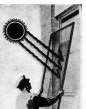
wire narrow as a pencil lead Vertical and paper-thin. wires spaced one-half inch apart hold the flat horizontals at a fixed angle, calculated so that it completely shuts out direct sun radiation during the heat of the day in all seasons. The mesh of the fabric is so fine one scarcely knows it is there at all.
