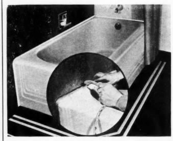
RUBBER moulding applied around bathtub with adhesive permanently seals this joint between wall and fixture.
