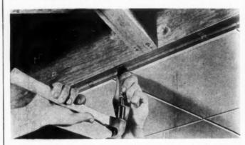
ABOVE illustration shows how a  $16'' \ge 16''$  Temlok De Luxe panel is erected directly to the ceiling joists, with two Tem-Clips being nailed in place against the leading edge of each panel. Prongs of the clips extend to grip the male edge of the next panel to be put in place. The workman is using the special magnetic head setting tool (furnished by Armstrong) which conveniently holds Tem-Clip and nail in proper position.
