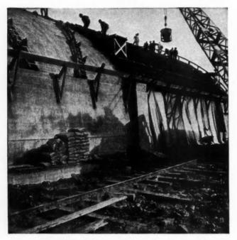
15,000 BARRELS of 'Incor' 24-Hour Cement, used in concrete roof of U. S. Navy Ship-Model Testing Basin, Carderock, Md., aided in completion six months ahead of contract date. About 60,000 bbl. of Lone Star Cement were also used.
