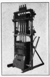
**AB214** The illustration above erated Stripper Cement Block Machine used in connection with the Miles Automatic Power Tamper, as developed by The Miles Manufacturing Co., Jackson, Mich. This is a combination of units that supplies a large production of high quality concrete blocks or tile at the minimum expense. Miles Automatic Feeding Units are available for use with the above machines for the purpose of supplying a still larger production.
