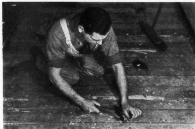
OLD floors should be repaired, tightened and smoothed, as shown above, to receive linoleum, or put over a hardboard base (below).
