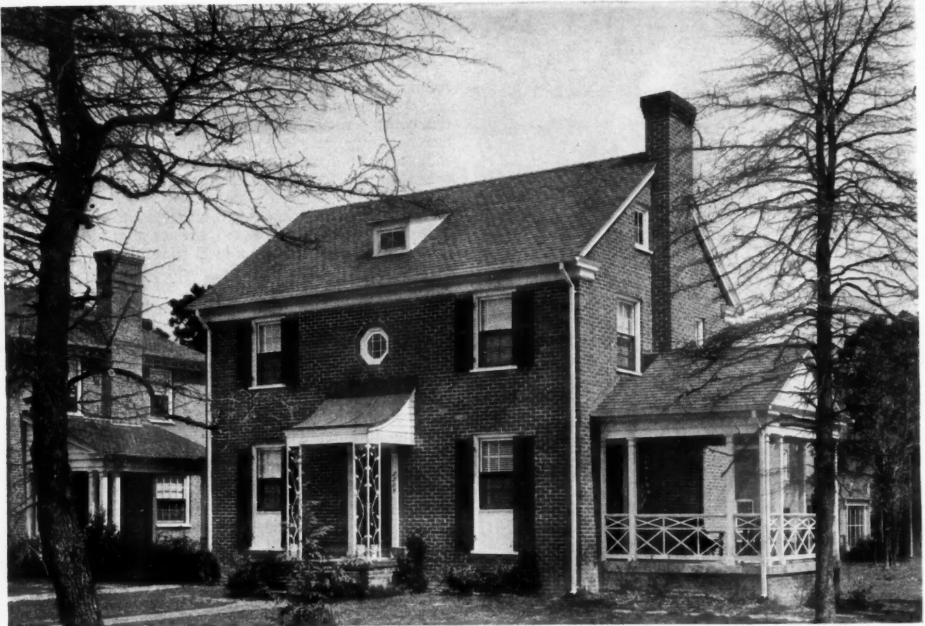
HAND-WROUGHT IRON WORK on front entrance gives unusual charm to this Matt. P. Will home in Glenburnie community at Richmond, Virginia.
