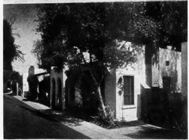
TWO VIEWS of Hollywood Terrace homes; note new fireplace chimneys.
