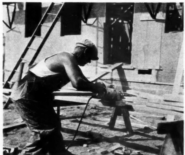
FAST electric power saw on the job handles miscellaneous cutting. The Whyte shop in Hackensack is completely equipped with woodworking equipment including saws, joiners and sanders.
