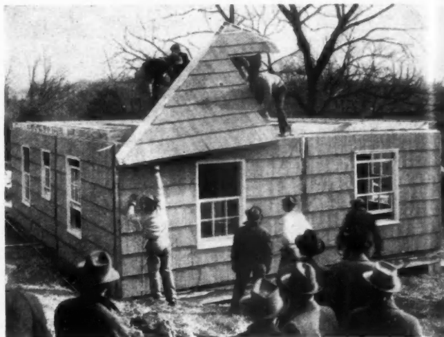
11:50; Gable-end panels placed.
