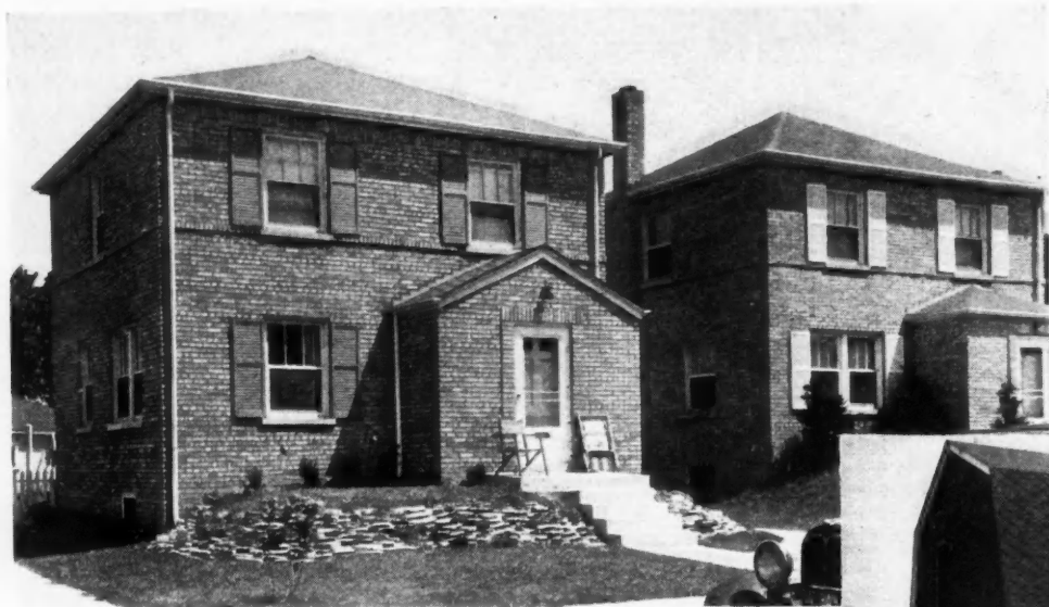
LEFT: Two of Builder Harry M. Quinn's basic 24' x 28' 6" six-room houses, with detail variations, built on 35-foot Chicago lots. Below, alternate style with same first floor and two bedrooms above as shown in the floor plans below.
