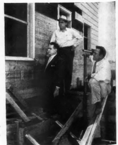
GROUP inspecting new C.A.C. unit window installation.
