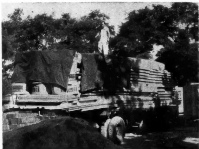
1—HUGE trailer truck delivers one complete story of apartment, including all floor and wall sections.
