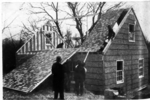
12:50; Roof panels go on.
