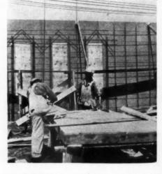
SHOWING the smooth surface of concrete, resulting from the use of Celotex Absorptive form liner on walls.
