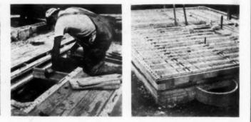
FOUR views above, left to right: Setting precast concrete floor joists; precast joist framing for first floor complete; inserting spreaders; and screeds in place for wood floor.
