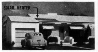
POPULAR Miami Shores home, with solar water heater frame on roof and water tank concealed in chimney.
