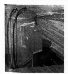
SOLAR water tank is built into chimney by Builder R. L. O'Dell. Electric booster unit heats water when sun doesn't shine.
