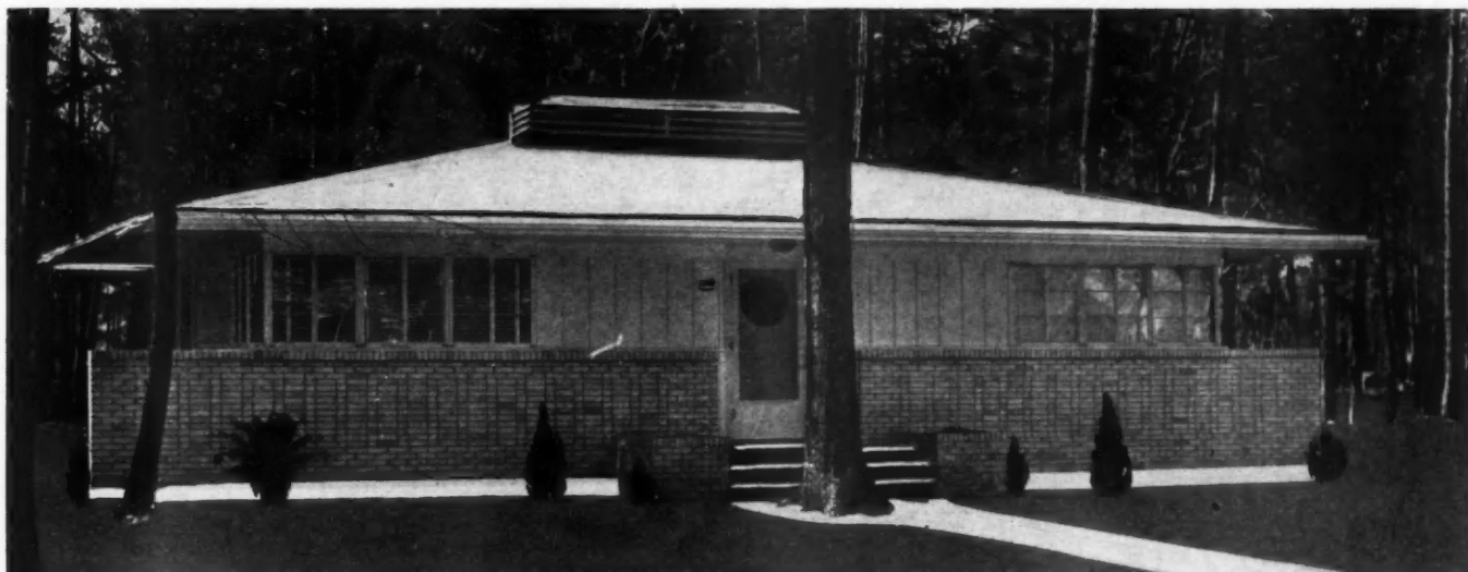
THE ABOVE Houston home, designed and built by the University Oaks Lumber Company, makes use of brick veneer for the lower portion of the front wall, with wings extending at the sides to align with the overhanging eaves. Vertical boards and battens break up strong horizontal lines.
