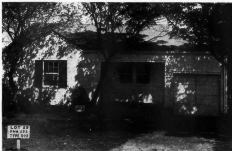
AN ATTACHED GARAGE has been added to this design, which otherwise is like Type A in number of rooms; all have fireplaces.
