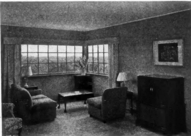
CORNER WINDOWS of living room command hillside view.
