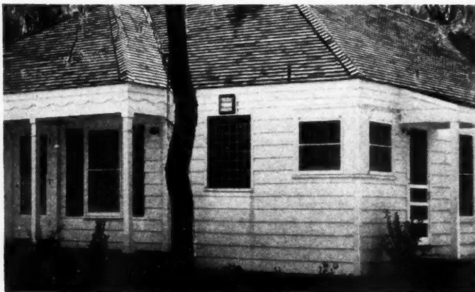
INSULUX panel in kitchen at front of house gives additional light, full privacy. Women like the easy-to-keep-clean advantages of INSULUX Glass Blocks.
