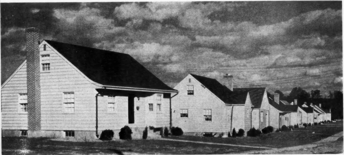
WORK IS BEING RUSHED on one hundred 31' x 25' defense homes for workers in nearby East Hartford airplane plants.
