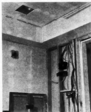
BEHIND-THE-SCENES wiring picture shows installation details of clock, doorbell and private house telephone system, which brings every room within arm's reach.
