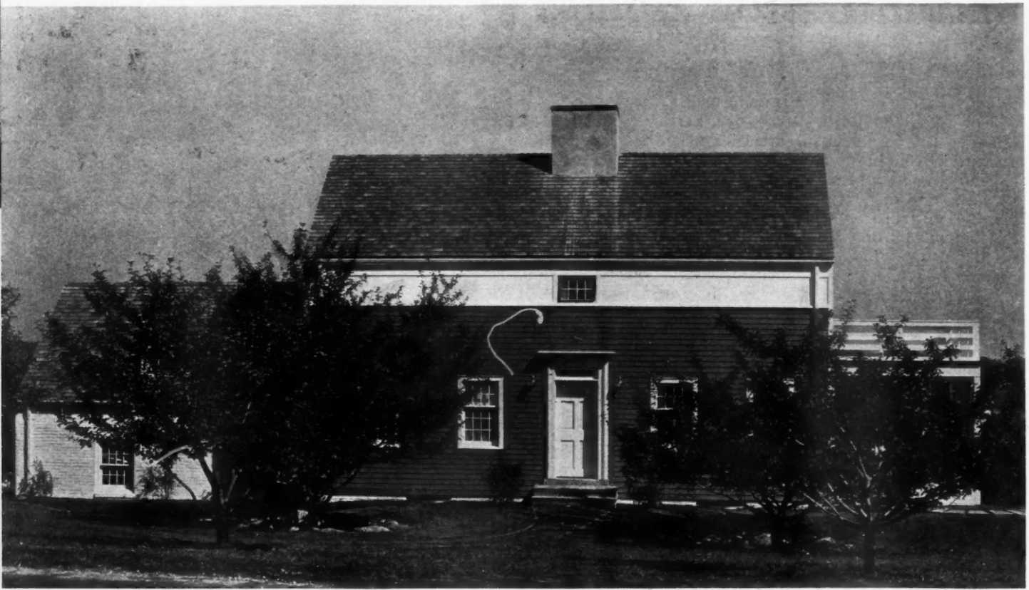
LARGE SMALL "HOUSE OF IDEAS" is designed in Early American salt-box style to fit sloping hillside. Victor Civkin, architect.
