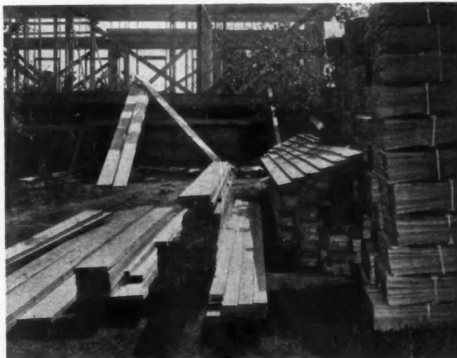
RED CEDAR SHINGLES, packaged siding, guide-line framing on job.
