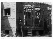
LARGE BOARDS of Temlok Lath are quickly and easily nailed to joists and studding. They provide efficient, lasting insulation, and a strong, firm, and permanent base for the plaster finish.
