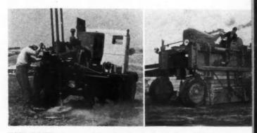
HOLE BORER was used to dig foundation holes. AT RIGHT-Huge carrier transports lumber from cars to prefabrication plant.
