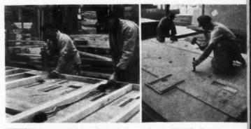
WIRING is inserted in wall sections at shop. RIGHT—Templates are used in cutting openings for outlet baxes.
