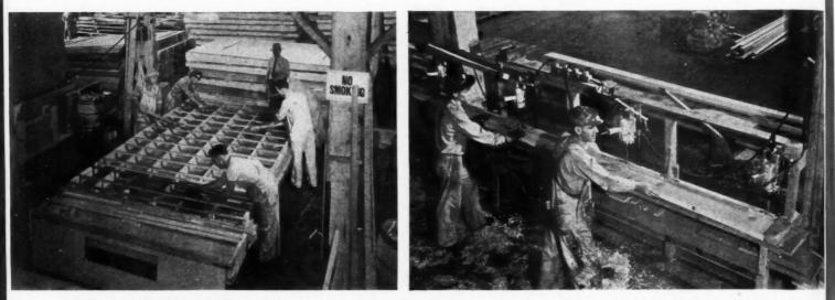
BUILDING CEILING SECTIONS—Building board is glued and nailed to furring strips on bottom of rafters. RIGHT—Multiple drill in operation—one of many types of power equipment that were used.
