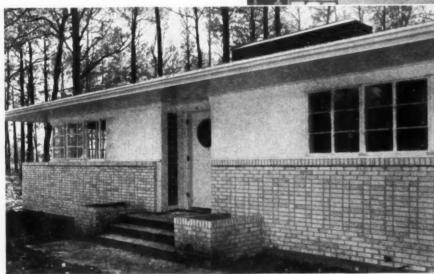
THIS Houston, Tex., home (plans shown in December '41 American Builder) has two Insulux block panels flanking the recessed entrance way. Here, light is the only consideration, and due to insulation value, fuel is saved. Below, a block panel lights the stairway in another Southern home.
