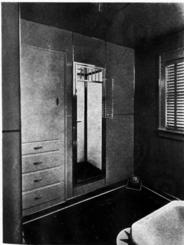
NEW bathroom showing "In-a-Wall" style of installation of cabinet shower, which is growing rapidly in popularity.
