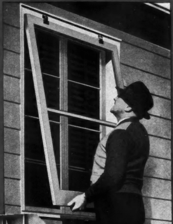
ABOVE—Simply hang ordinary storm sash atop, on outside of Fenestra Package Window. Storm sash not supplied by Fenestra.
