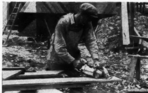
SAWING SIDE SHEATHING to measured angle cuts with Black & Decker Saw. These fast saws make any cut a hand saw will perform faster and easier.
