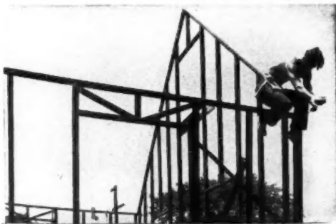
Frame units are fastened together quickly and easily with an ordinary screw-driver, using self-threading screws. Roof channel plate and wall-section channel plate are being assembled here.
