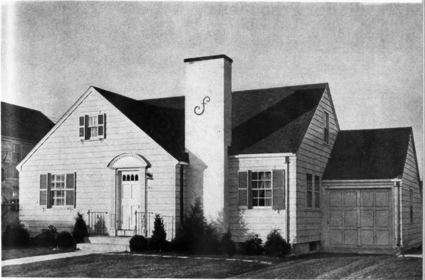
FRONT COVER war-worker home has fine architectural appeal and practical plan, as shown below. Main foundation is 34'-10" x 27'-10". Vestibule-stair arrangement good. Keith Sellers Heine, architect.
