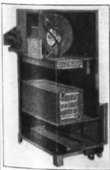
A PHANTOM view of vertical unit equipped with humidifier pan and water coil.
