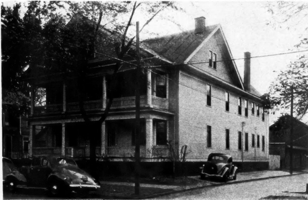
MULBERRY Apartments, Toledo, O., remodeled to make twelve small modern family units out of four large old ones. New apartments in demand by war industry workers.
