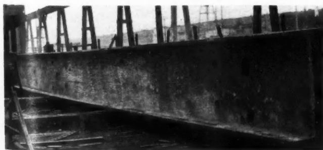
Fig. 2—The I-beam, which originally had been bent sideways 6 in. out of line, is shown here after it had been straightened by repeated applications of heat, followed by cooling. Total time for straightening was only 2 hrs. A second I-beam, similarly damaged, was straightened in the same manner.
