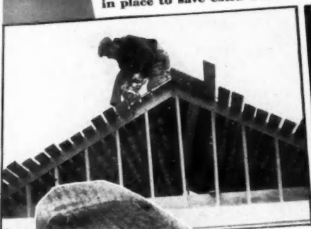
SKILSAW trims roof sheathing faster... after it is nailed in place to save extra time.
