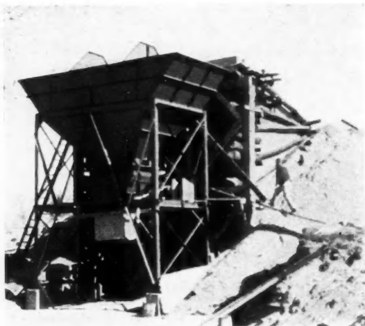
78-TON, 3-bin batcher used at Milbrook Park. Three ready-mix trucks deliver transit-mixed concrete to houses.
