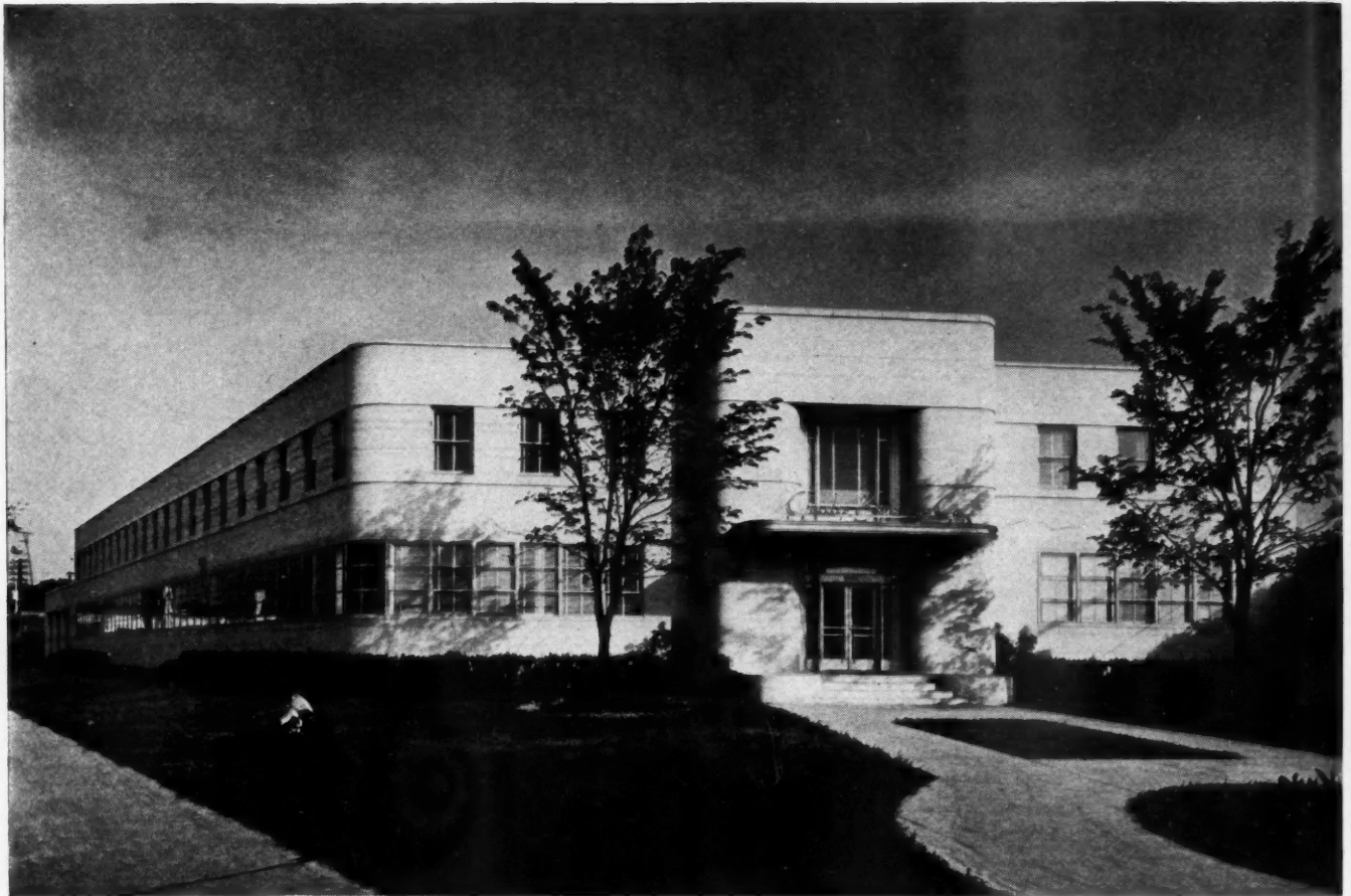
NEW PLANT of Charles Bruning Co., Inc., Chicago • ARCHITECT: Victor L. Charn, Chicago CONTRACTOR: B-W Construction Co., Chicago
