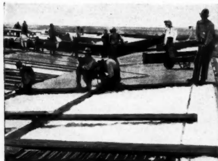
The steel roof deck was erected immediately after
