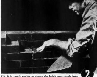
(1), it is much easier to shove the brick accurately into place, with a full head-joint, than it is to do the same thing with the other mortar (2).
