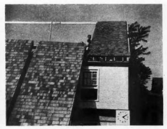
SHINGLED roof sections being moved into place.
