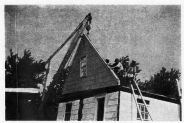
COMPLETE END-GABLE with window is set in place with crane.
