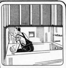
4. CLEAN GLASS and fill joints carefully with pointing compound supplied. This assures thorough waterproofing.
