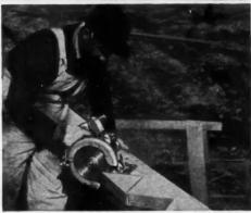
CUTTING stair carriages with Black & Decker Electric Saw takes only 35 minutes for a set of 3 carriages—compared to the cost of a half day's work when done by usual hand-sawing methods.
