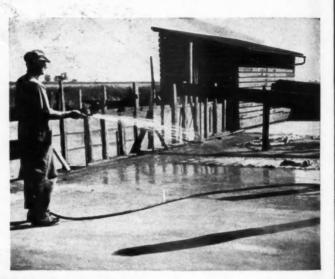
THE NEW concrete floor must be protected from drying out for at least 5 days by sprinkling and covering with sand or canvas. The forms for a concrete manure pit can be seen in the background.
