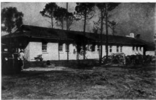
• Newly completed U. S. Army Mess Hall. This use of stucco made with Atlas Waterproofed White cement saved critical materials—lead, zinc and steel.
