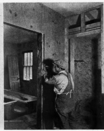
AIR DUCTS are run between joists and are of gypsum board, thereby saving on sheet metal; front hall is finished in Knotty Pine Sheet-rock, square edge boards butted tight to make an invisible joint.
