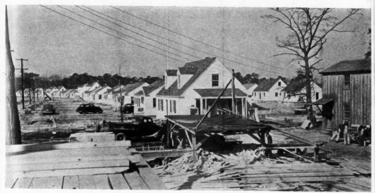
FOUR HUNDRED houses are scheduled by Contractor V. T. Myers in his Monticello-home job in Norfolk. Lumber stored in foreground is pre-cut on power saw, trucked to each foundation site. BELOW: Red cedar shingle exteriors being applied. Plans on next page.
