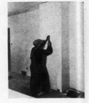
NAILING up gypsum wall lining with the new wider nail spacing 6" apart.
