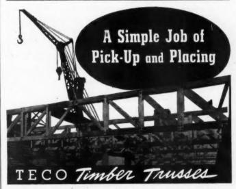
The TECO Timber Trusses used on this 50' x 225' truck garage were assembled on the job and quickly hoisted into place by a gasoline crawler crane.
