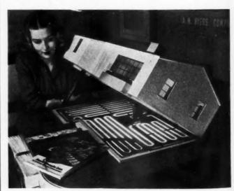
MODEL house tips up to show heating pipes in floor.
