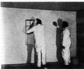
BIRD "Monacousec" is applied to walls horizontally over uncased openings, which (as illustrated below) are afterwards cut out, and the finish surface washed.
