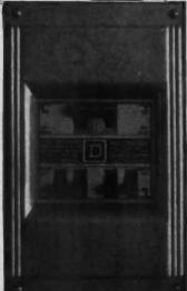
Here is the type of Multi-breaker used in the "Miracle" homes. It provides for a range circuit and four lighting circuits.
