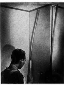
EXTRUDED Tenite strips for covering wallboard seams and joints are easy to apply. No nails, adhesives, or painting are required. The strips are so shaped that they become automatically secured when forced into the seams.
