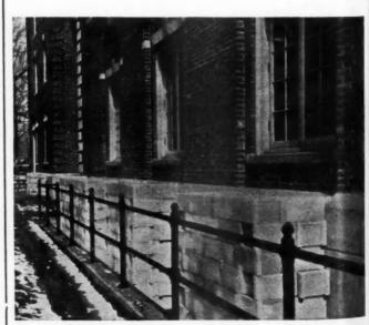
HOLLOW 12-in, concrete masonry units laid up without mortar are used to protect basement windows in dormitory building at Radelli College, Cambridge, Mass., prepared for use as a bomb shelter.
