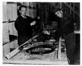
SWITCH BOXES, outlets and coils of wire cable are attached to studding in electrical workshop. These studs are then built into wall sections with wires protruding, ready for quick connection at site. All wiring operations have been highly standardized and greatly simplified.
