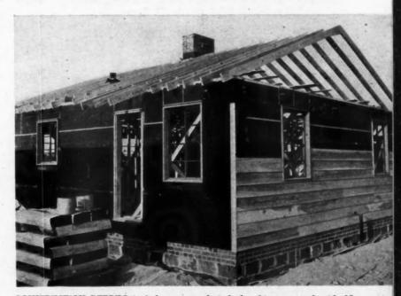
CONSTRUCTION DETAILS include gypsum board sheathing covered with 15 lb. felt, well lapped. Thick-butt asphalt shingles, piled in foreground, are used on roof. Roof ratters are  $2 \times 6$ , with  $2 \times 6$  ceiling beams. Houses have 2'' of mineral wool insulation in attic floor.
