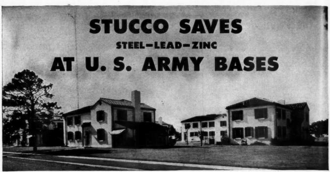
Durable buildings of concrete block or cinder block or clay tile, finished with white portland cement stucco or white cement paint, provide good construction and save materials and transportation essential for war.
