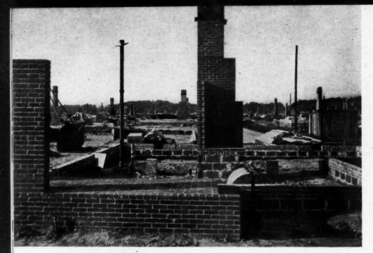
A FOREST OF CHIMNEYS rises from the site of the Levitt job as more than 300 foundations are completed before carpenters come on the job. Rough plumbing was installed first.
