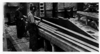
BUILDING END GABLES on special jig table. Redwood siding is nailed direct to 2 x 3 studs covered by 30-lb. felt.
