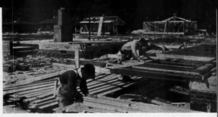
APPLYING SIDING to exterior wall in horizontal position. Doors and windows are installed and wall is completed before raising.
