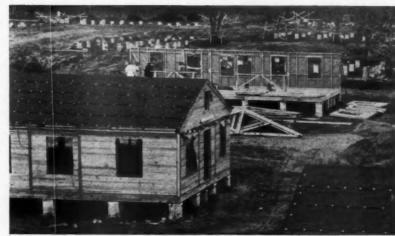
CONSTRUCTION VIEW showing units in various stages; panels are shown being erected; piers for other units seen in background.
