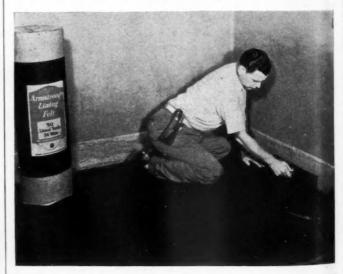
HERE a mechanic is applying Armstrong's new semi-saturated lining felt to be followed by linoleum.
