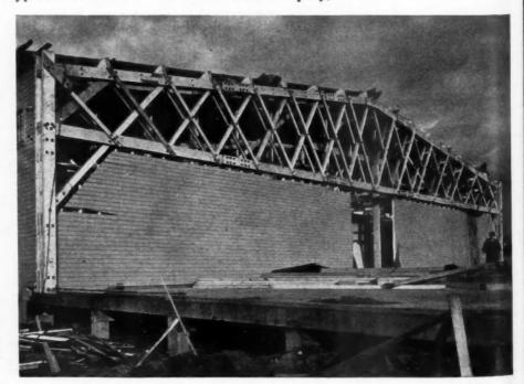
AT TOP of page: Interior view of Pacific Forest Industries enlarged warehouse showing Teco connector wood trusses. Right: End of building where addition was made: new piers, joists, flooring and first truss in place.
