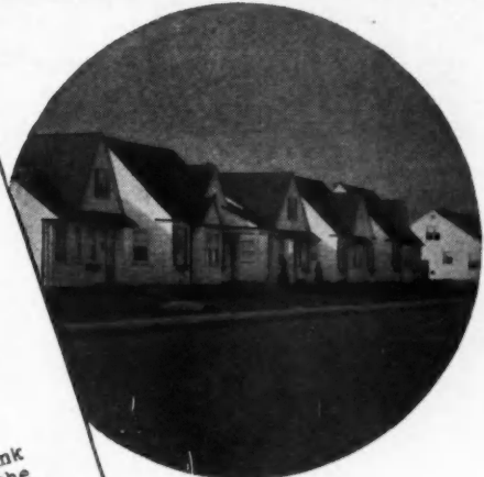
Another view of the Rosedale Gardens Project
