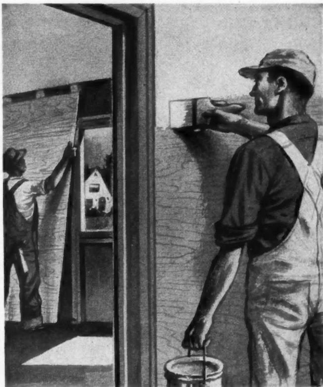
Weldwood Utility Paneling makes strong, rigid walls. With nailed and glued invisible butt joint it forms an ideal base for paper or paint.
