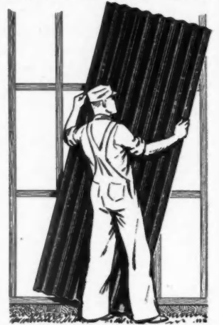
CORRUGATED asphalt siding.
