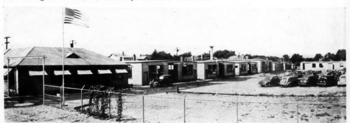
CRITICAL MATERIALS CONSERVED in this new plant for The Ready-Power Company, Detroit, Michigan, Eight wooden unit buildings, each 60' x 80', give required floor space, light, air, and break up fire hazards.
