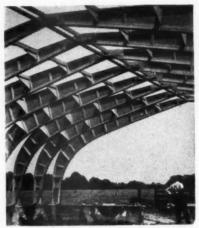
PLYWOOD ARCHES for naval buildings, airplane hangars, barns, etc., have plywood arch beams for strength and unobstructed floor area—new handbook
