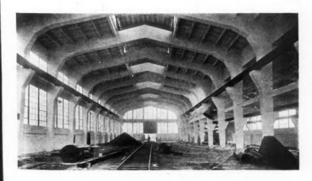
AT the left is shown a heavier type of concrete construction in a plant suitable for turning out larger pieces of war equipment. A heavy-duty floor is required in this case.
