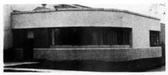
PICTURED ABOVE is the kind of plant addition which will be required in enlarging industrial facilities for war work where more space is needed for an engineering department, administrative office, etc. The details at the left show concrete masonry construction applicable to this and to numerous other plant expansions.
