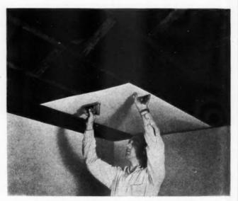
WORKMAN applying Carey Asbestos heat duct.
